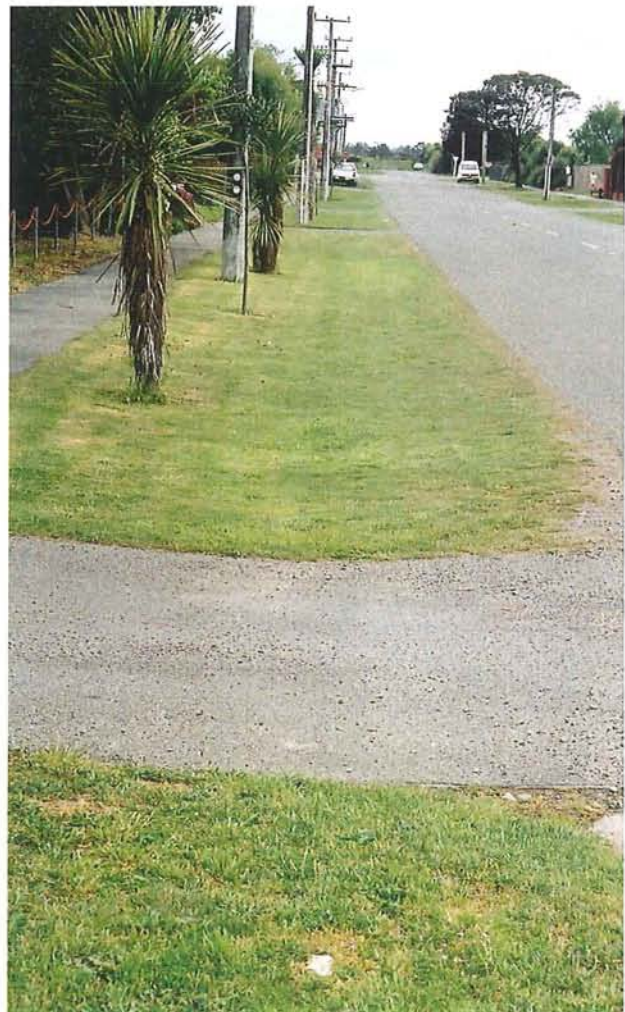
Figure 5-2: Cutting the grass too short in vegetated swales, such as illustrated above, will reduce the efficiency of the swale. For peak efficiency the swale needs a dense mat of vegetation. Lower Styx Road, Brooklands.
