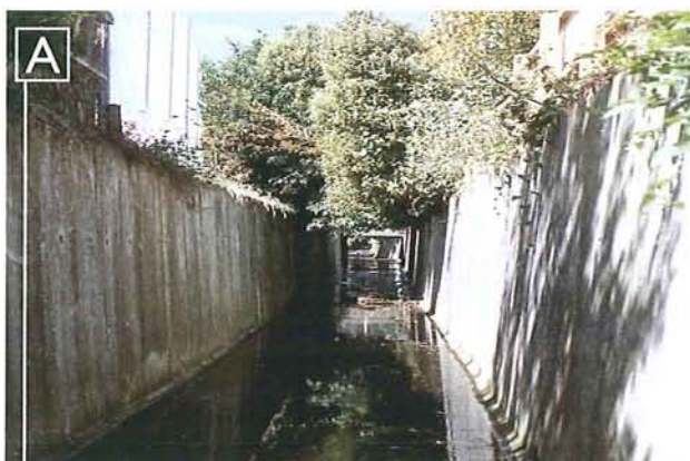
Figure 2-5A: Concrete lined drains were once installed for good drainage, and to prevent erosion caused by increased flows following channelisation. Victory Drain at Centaurus Road.
