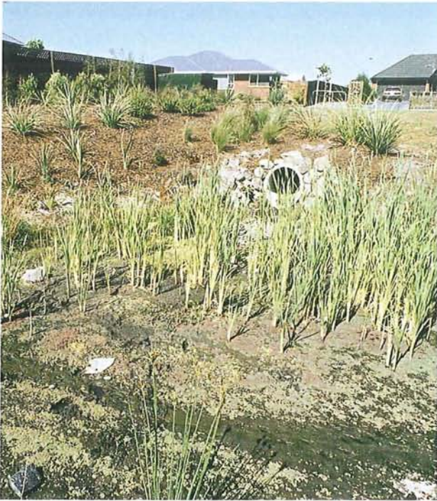
Figure 14-6: This low outfall was terminated back from the stream and the area planted in rushes. The rushes now hide the outfall from view. Kaputone Creek, Sheldon Park.
