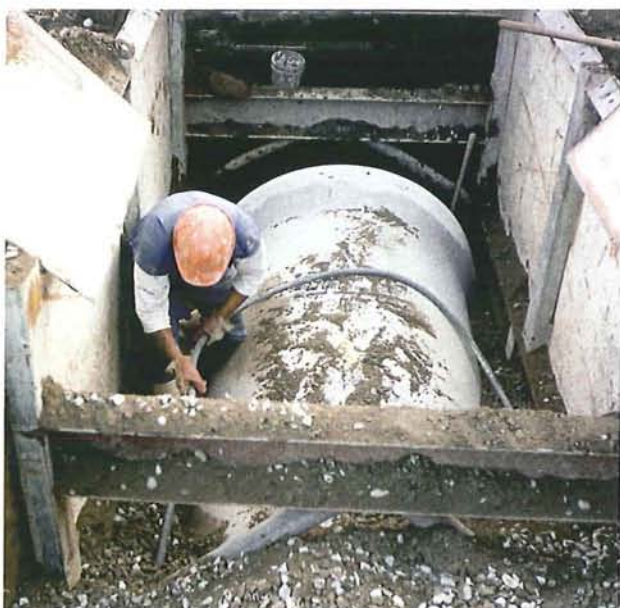
Figure 14-2: Laying of a 1200 mm stormwater pipe, Wilderness Drain.
