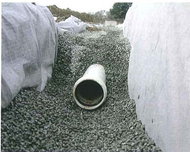
Figure 14-1: Laying of a 175 mm roading related stormwater pipe.
