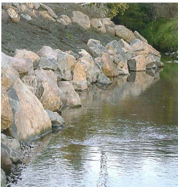
Figure 12-4: Rocks of two to three levels backfilled with gravel can be used for a stone wall. Try to ensure the rocks do not create a uniform edge, but have some 'nooks and crannies' at the water's edge to provide instream habitat.
