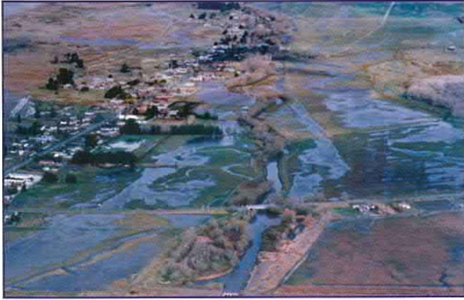
Styx River flood plain, Brooklands - storm event 1992 Opposite: floodgates, Styx River near Harbour Road
