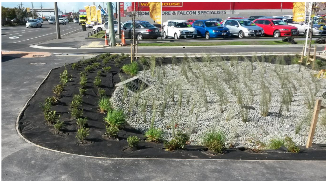
Figure 35 Rain garden media contoured to form ponding area.
