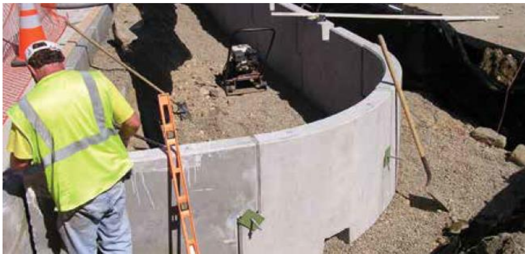
Figure 21 Precast concrete walls allow for fast installation
