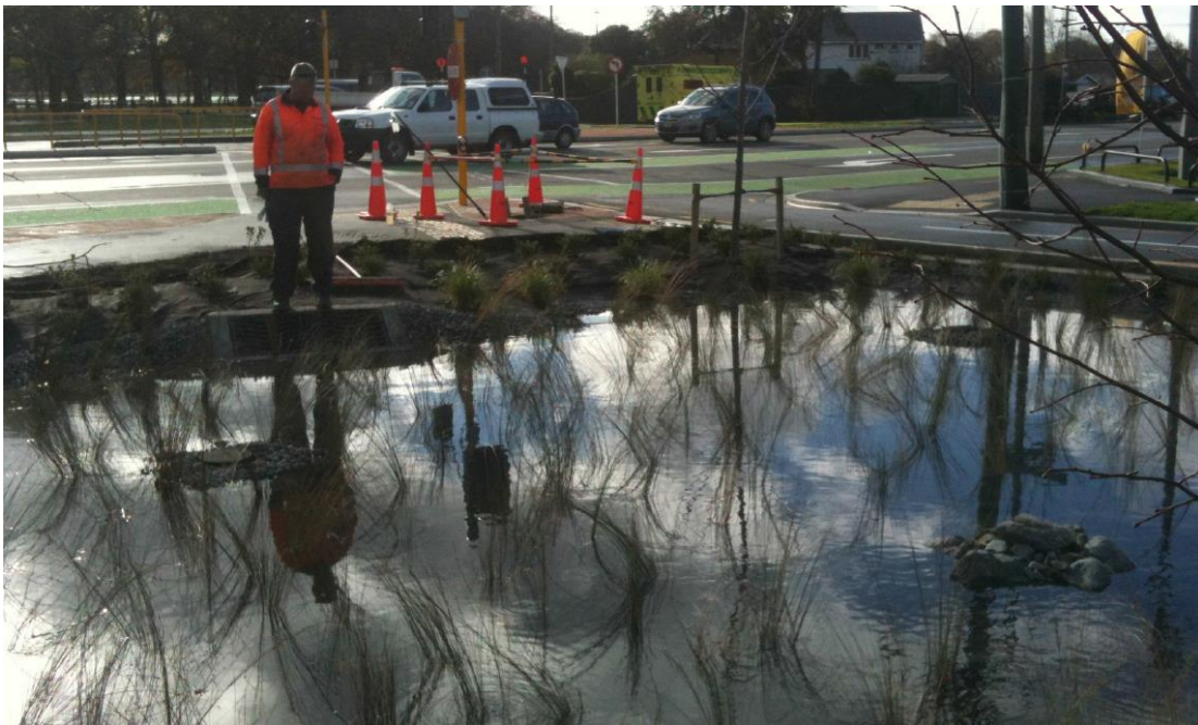
Figure 30 Grove Rd rain garden during infiltration testing
