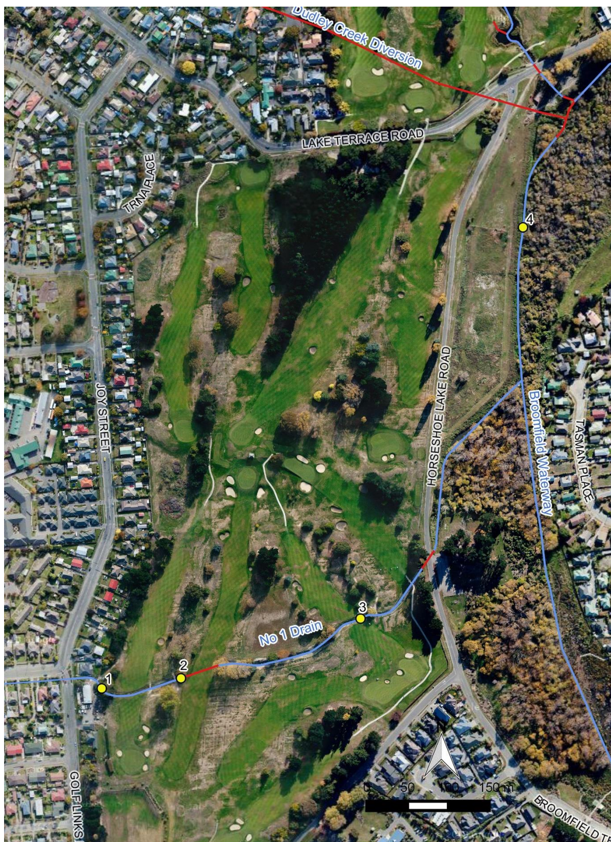
Figure 1: No. 1 Drain and ecology sampling sites (numbered yellow circles). Blue lines indicate open waterways, while red lines typically indicate piped or culverted sections. Satellite Imagery from Google.
