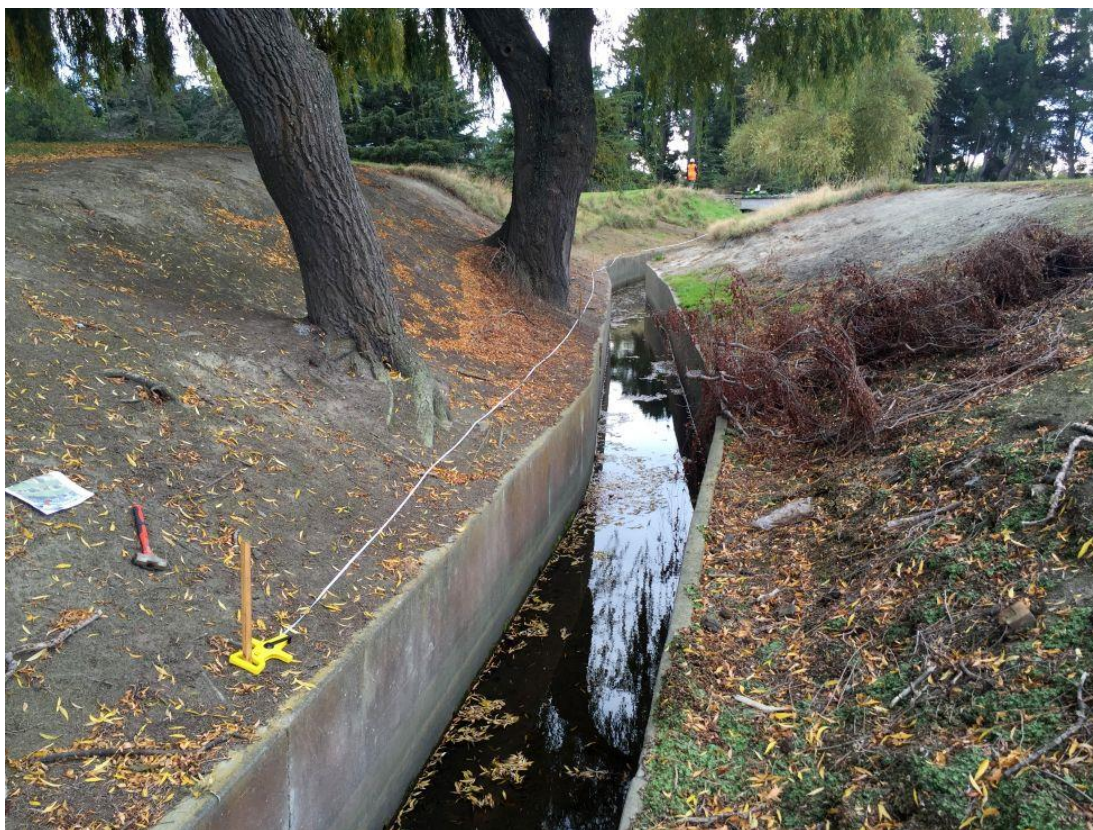
Figure 6: Site 3, view downstream from the top of the reach.
