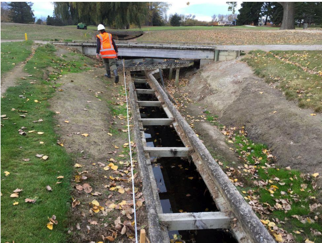
Figure 4: Site 2, view downstream from the top of the reach.
