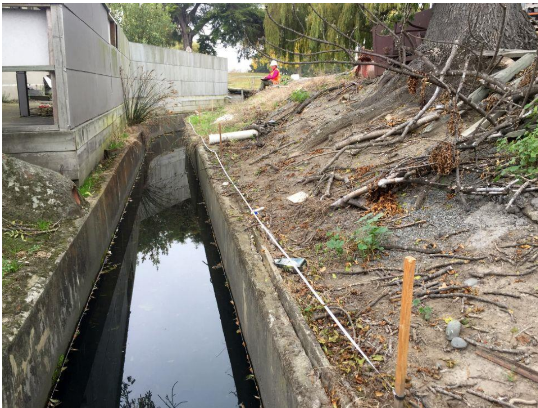
Figure 2: Site 1, view downstream from the top of the reach.
