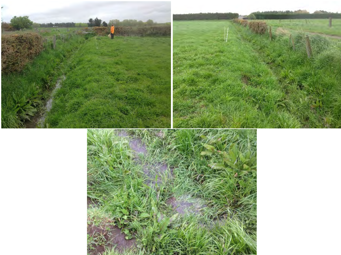
Photo 4. Site 4: Days Waterway – downstream, located approximately 250 m upstream of its confluence with Henderson Waterway, looking upstream (top left) and downstream (top right), looking into the channel (bottom).
