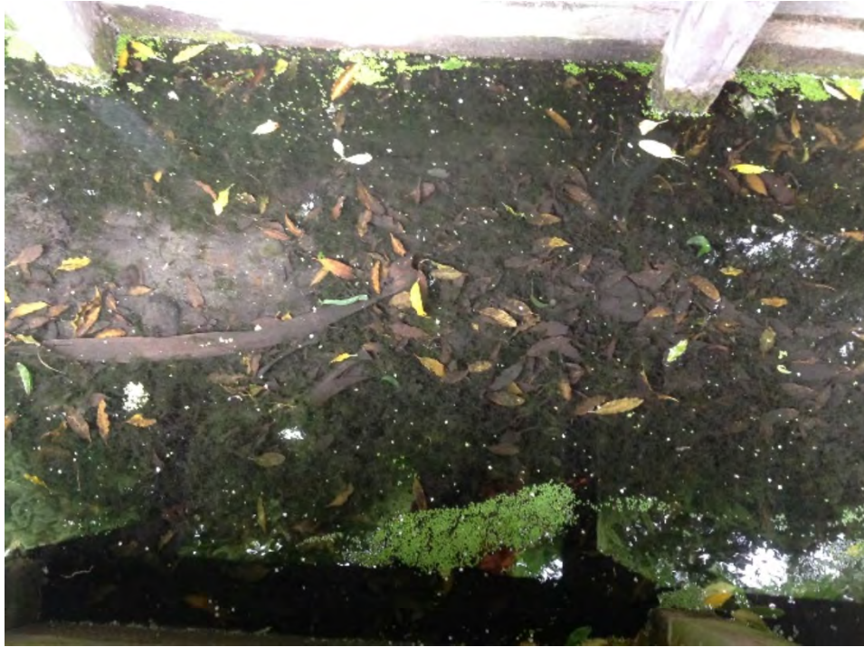
Site 5: Hendersons Road Branch Drain, November 2016
