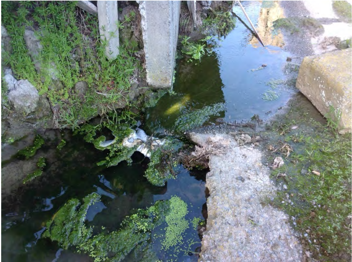
P3: Perched concrete sill, which may be a barrier to fish passage during periods of low flow, downstream of Site 4 in Days Waterway.
