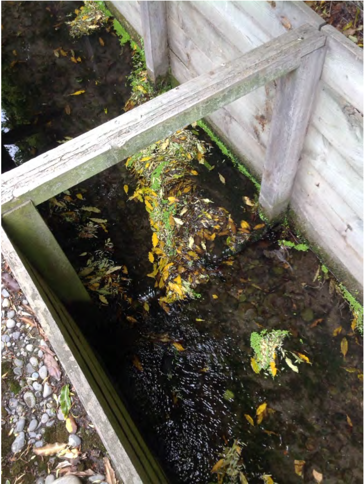
P2: Timber cross beam may be a barrier to fish passage at times of low flow; Hendersons Road Branch Drain, approximately 20 m downstream of Site 5.
