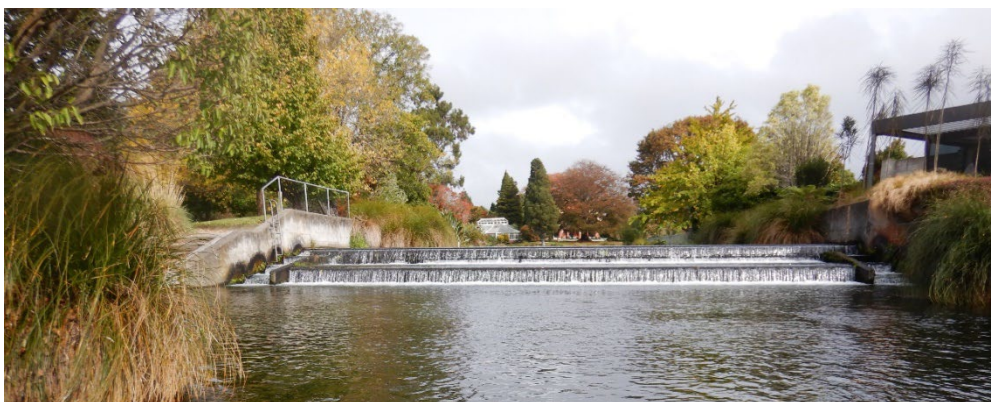
Figure 1. Looking upstream at the Mona Vale Weir (Weir A) pre-remediation. A trout ladder was constructed on the true right bank but still presented a barrier to salmonids.
