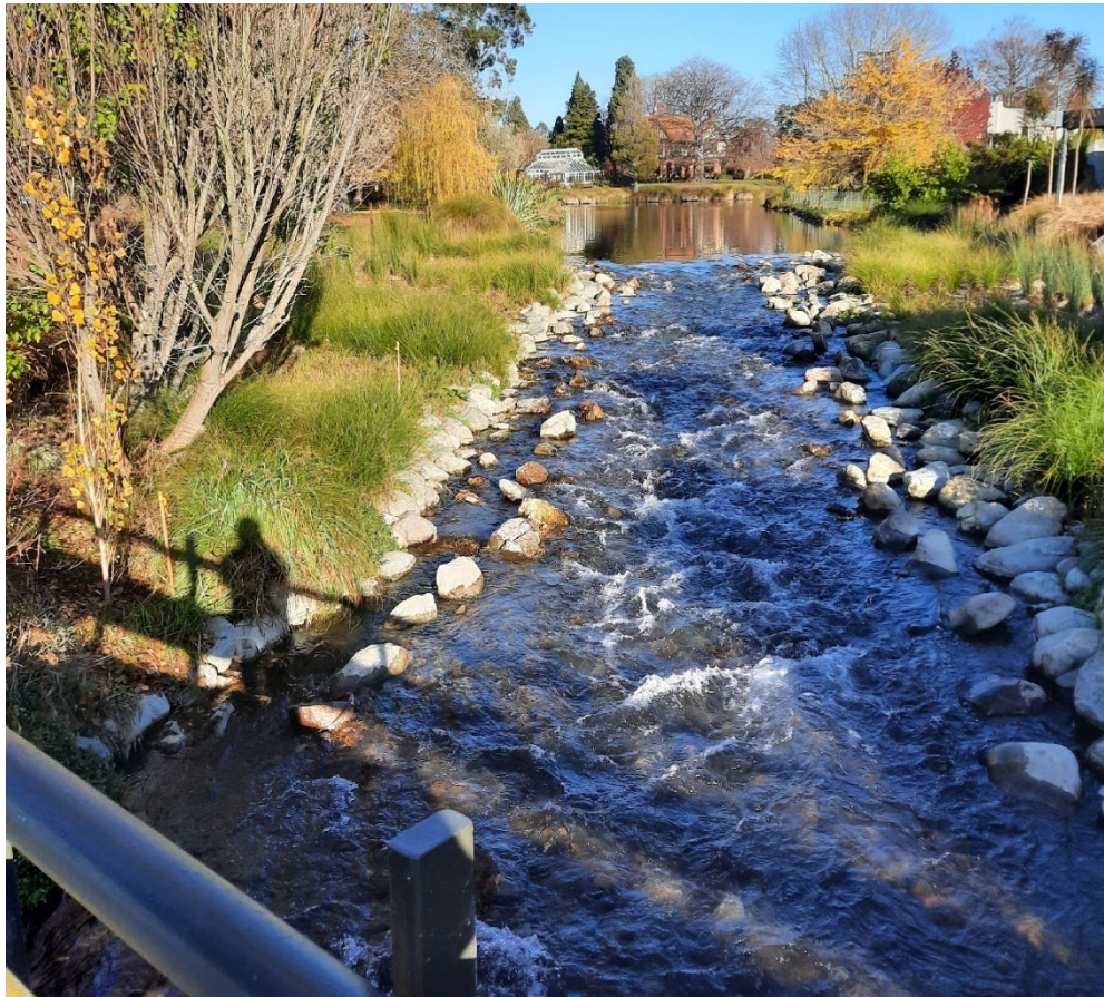
Figure 2. Looking upstream at the constructed rock riffle (Weir A) post-remediation.
