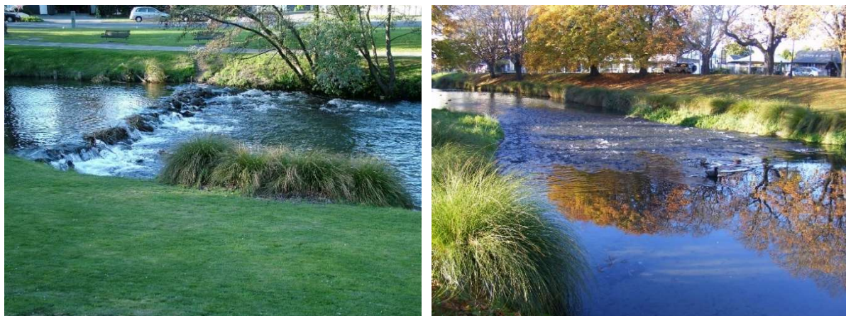
Figure 9: The unstable rock weir (left) and the replacement rock riffle weir (right).
