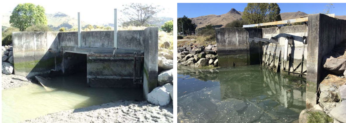
Figure 14: The old tide gates (left) and new fish friendly tide gates (right) in Avoca Valley Stream near the Ferrymead golf course.
