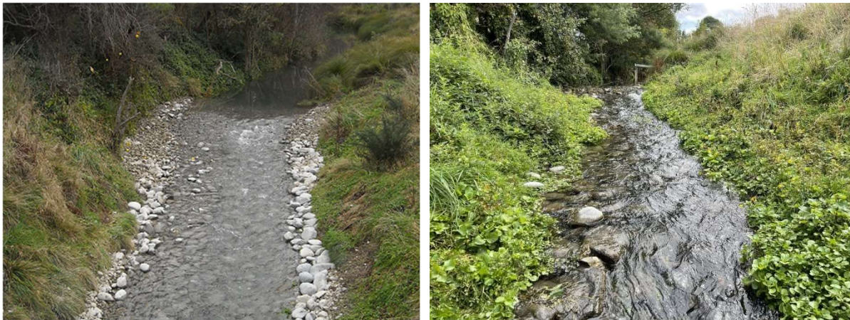
Figure 16: The weir just after construction in 2015 (left) and in 2021 (right).
