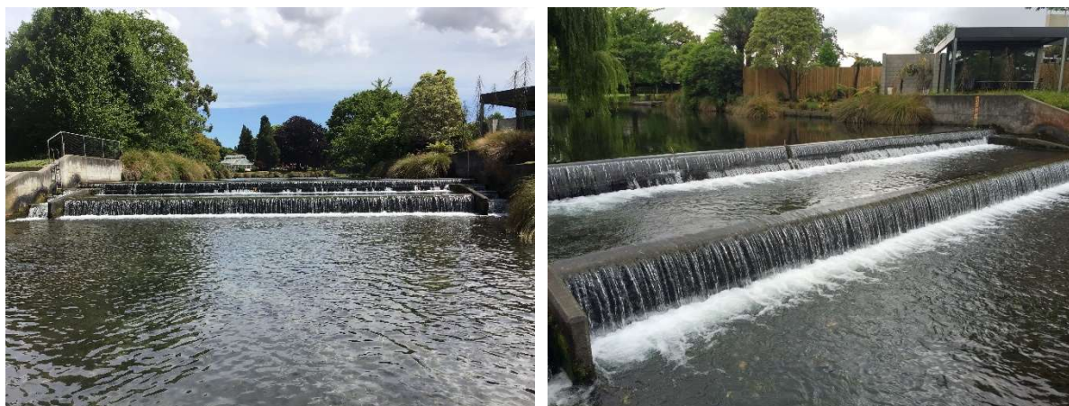
Figure 10: Photographs of the weir in the Avon River at Mona Vale.
