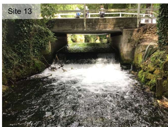
Figure 8: Four weirs on the Avon River that are the highest priority for improving fish passage of the structures assessed. The structures are located near Mona Vale (Sites 11 and 12), Christchurch Boys High School (Site 13), and downstream of Clyde Road (Site 14).
