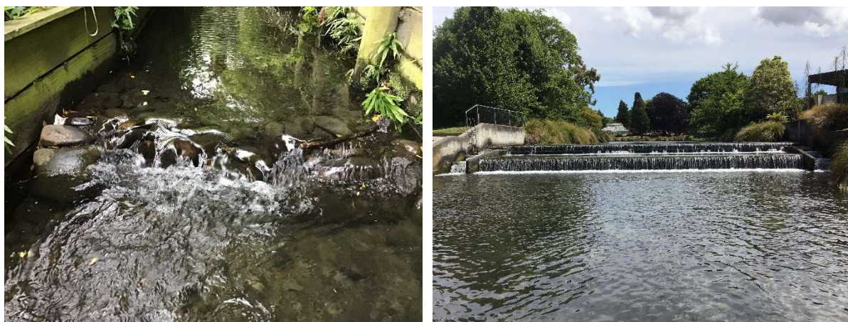
Figure 4: A low-level weir made of rocks (left, Site 20) was qualitatively assessed as a medium risk to fish passage, but had an FPAT assessment of very high risk. A large weir on the Avon River (Site 12, right) was considered a high risk by both methods.
