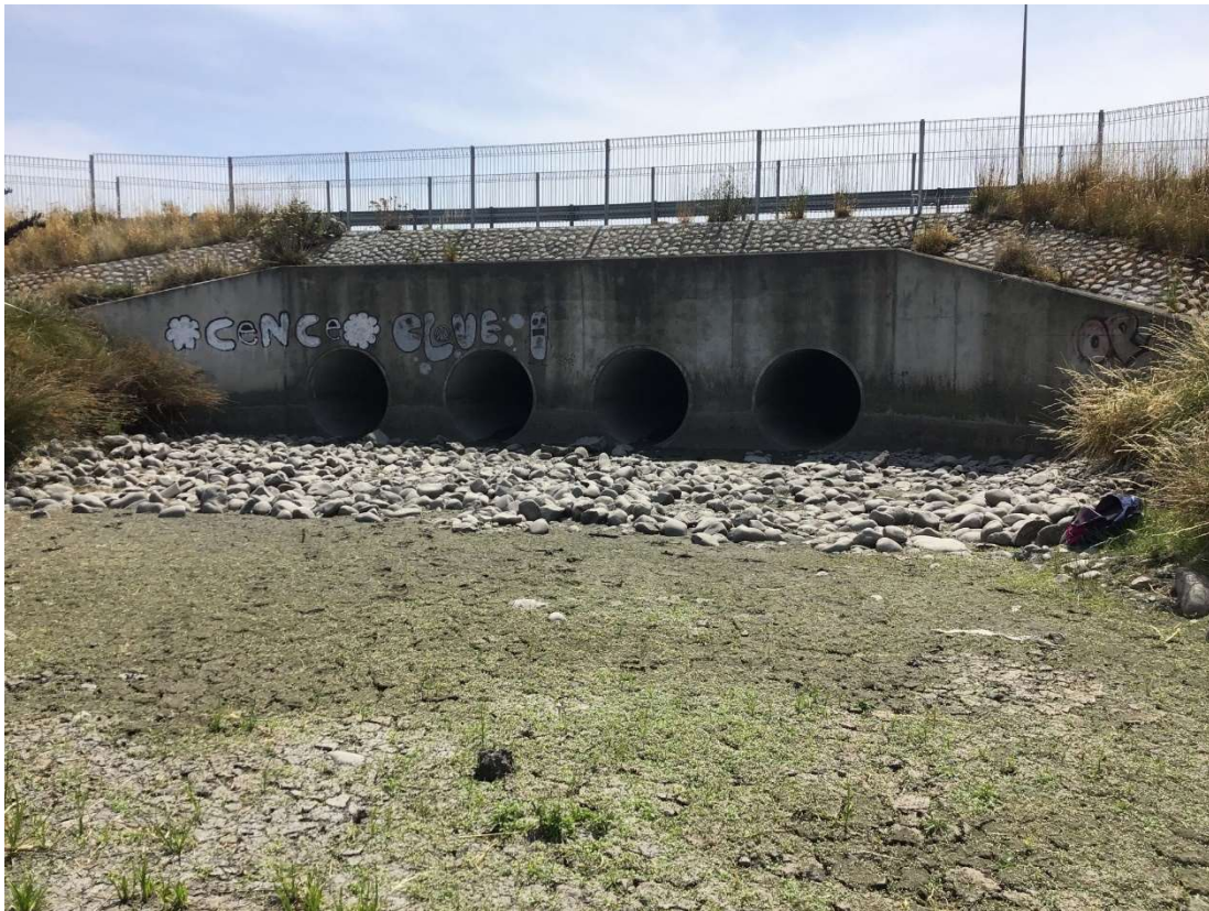
Figure 33: Site 36 (downstream end).
