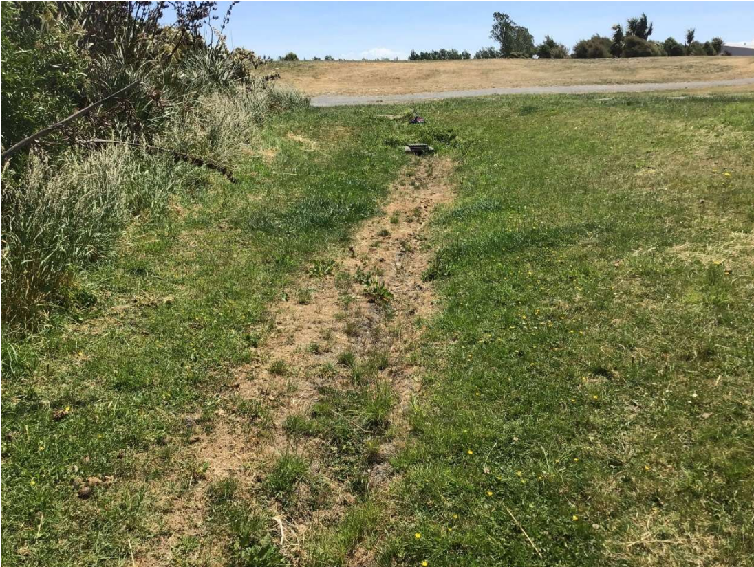
Figure 5: Site 6c (downstream end).
