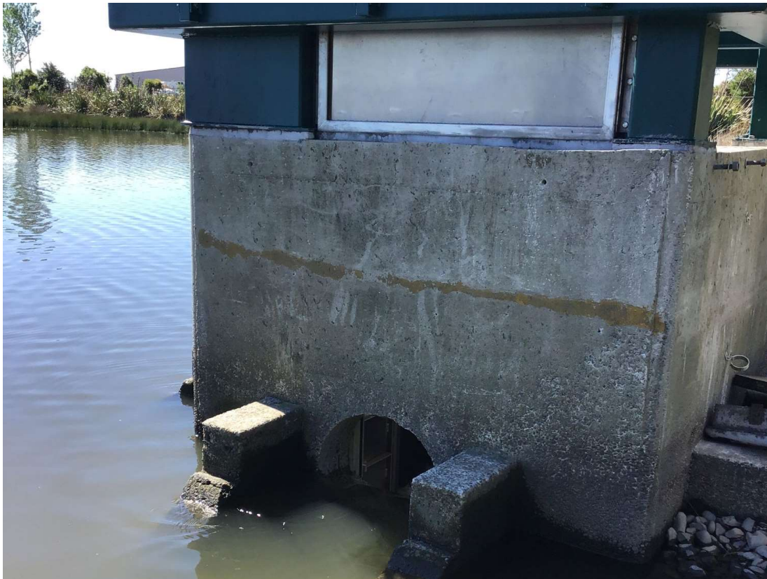
Figure 3: Site 6a (upstream end).
