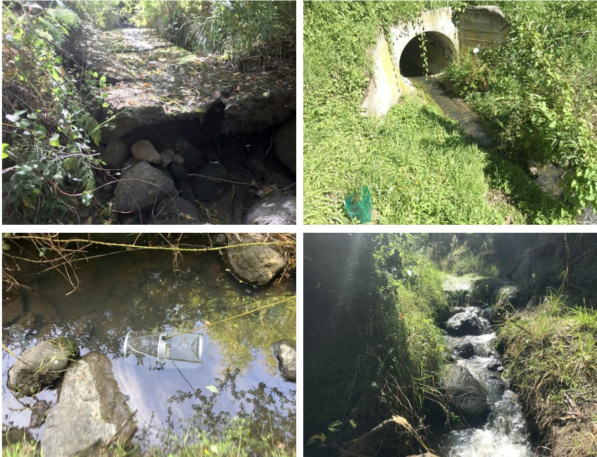
Figure 10: The perched apron at the downstream end of the Omaru Stream culvert (top left), the upstream end of the culvert (top right), a pool typical of the reaches sampled downstream near the Rāpaki Marae (bottom left), and the Upstream 1 sampling reach.
