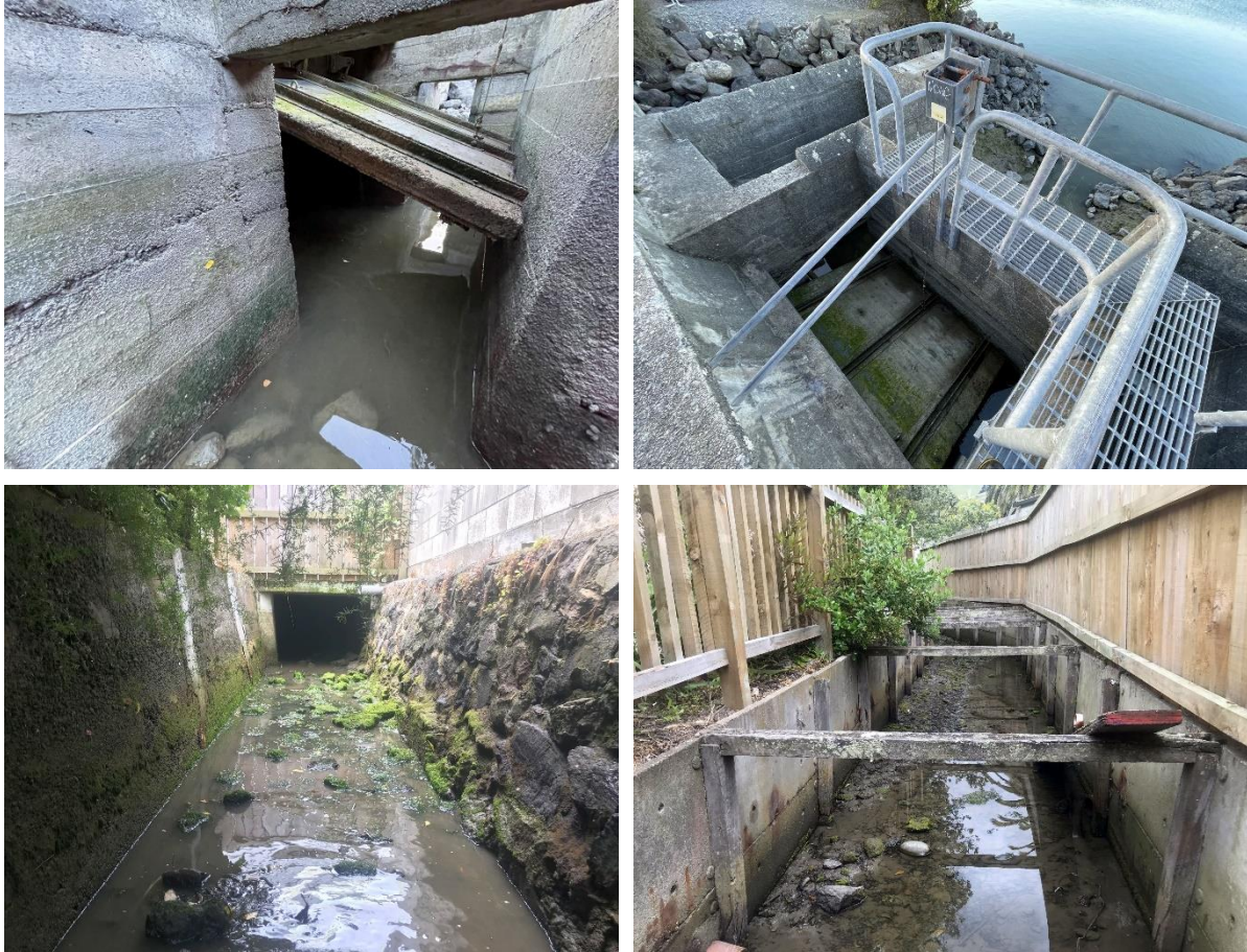
Figure 7: Rifle Range Waterway, including the flap gate outlet (fixed in an open position; top) and the habitat immediately upstream (bottom).
