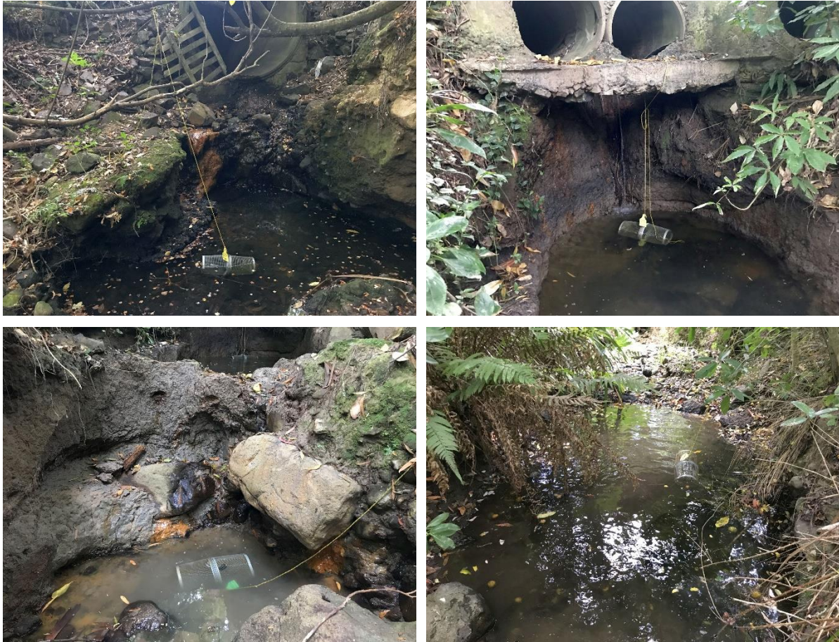
Figure 12: The perched culvert in Church Lane Drain immediately under Main Road (top left), a perched private culvert under a driveway downstream (top right), a natural barrier immediately downstream of the private culvert (bottom left), and the habitat sampled at site Upstream 1 (bottom right).
