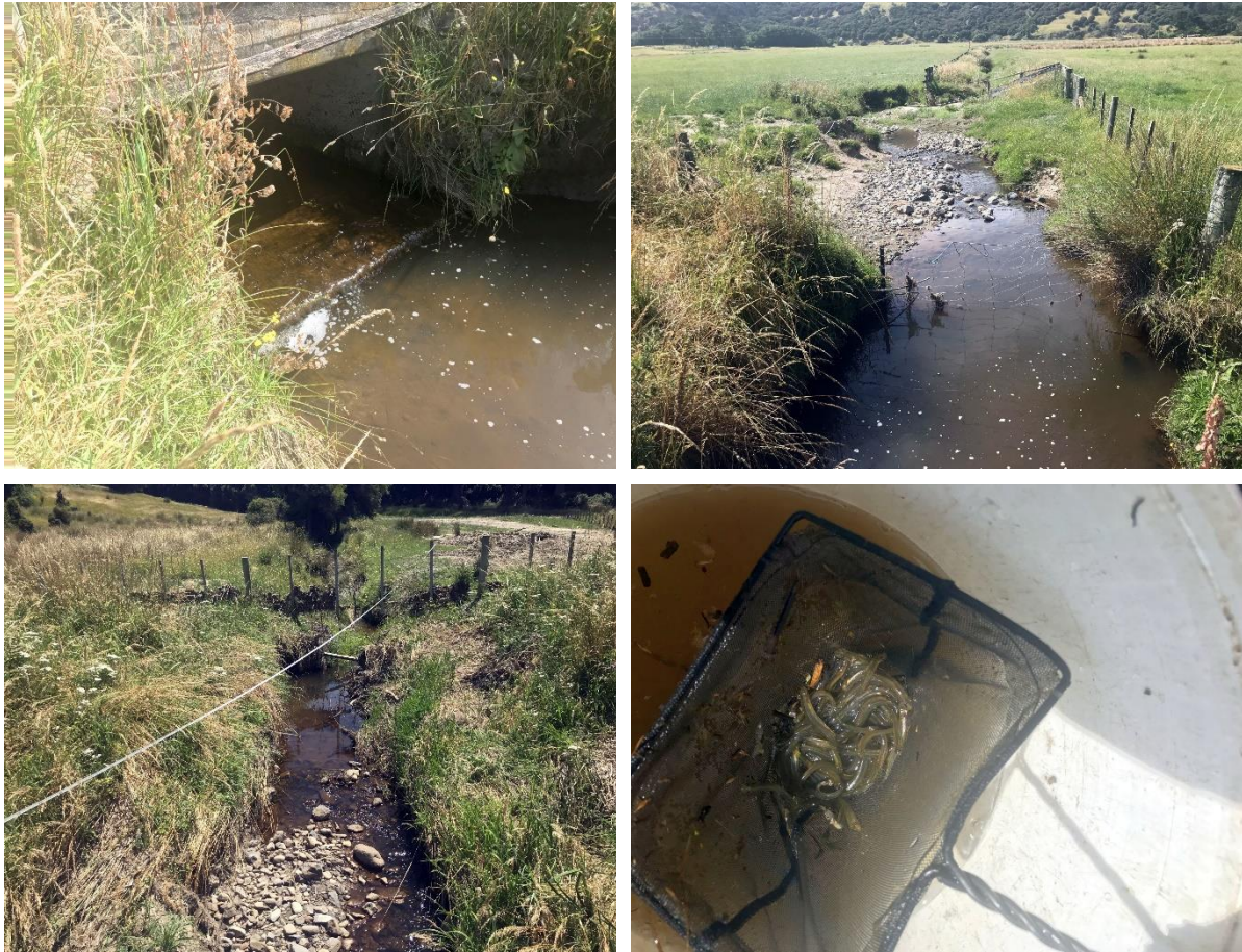
Figure 16: The slightly perched culvert in Le Bons Bay Stream Branch No. 13 (top left), the downstream sampling reach (top right), the upstream sampling reach (top left), and a photo of some juvenile galaxias (bottom right), which were caught both upstream and downstream of the culvert.
