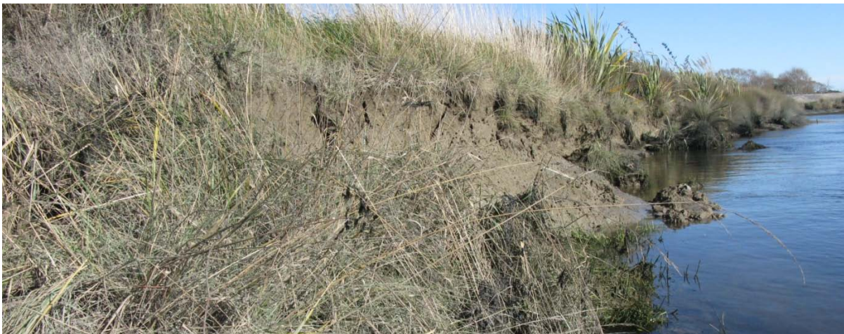
Figure 29. A large section of bank of the lower Styx River appears to have collapsed recently. There is no stock in the area, nor walking tracks.
