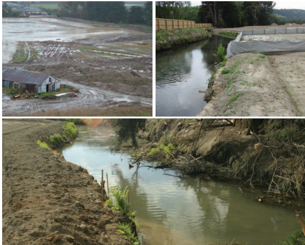
Figure 6. Sources of sediment input into Cashmere Stream during land clearance (top left) and bank works for the new subdivision off Penruddock Rise. Some sediment control measures were used for stormwater runoff sites (top right) but in other areas loose soil was pushed over the bank's apex and rolled into the stream (top right, above).
