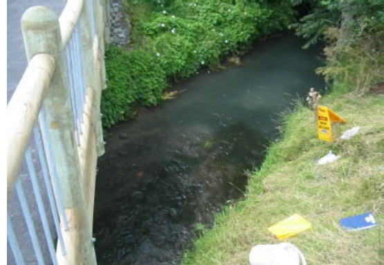
Site 1: 2005 Survey: Immediately downstream of Cashmere Road bridge, looking downstream from foot bridge. (Note the new footbridge to the left of the image).
