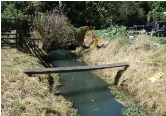
Site 3: 2007 Survey: Upstream of Dunbar's Drain, looking downstream.
