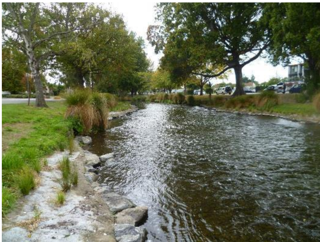
Photo 17: Rehabilitation Site 5 looking downstream
