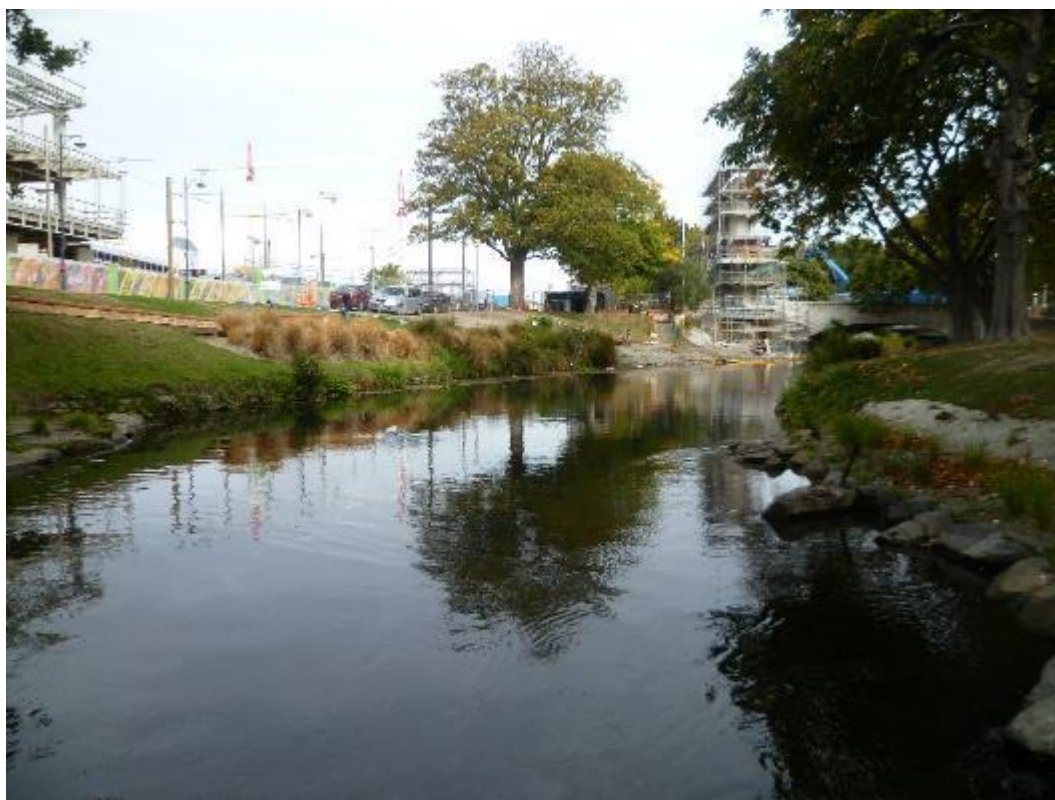
Photo 13: Rehabilitation Site 3 upstream of Hereford Street Bridge, looking upstream
