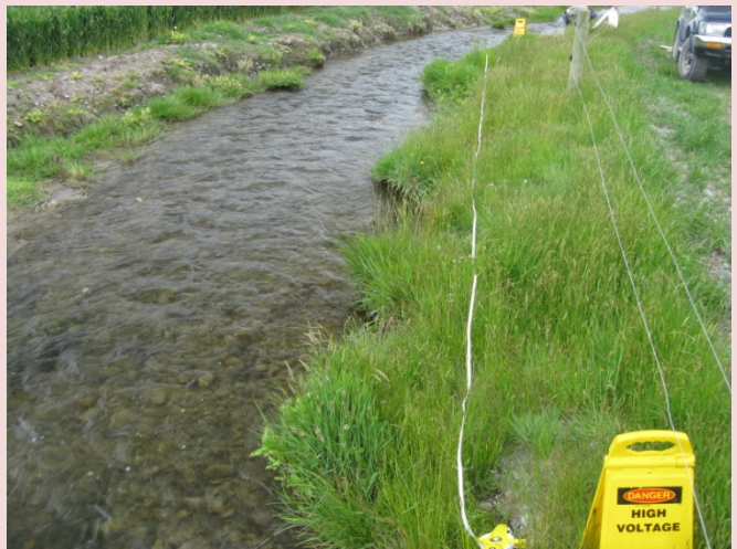
Figure ii(b). North Boundary Stream, Site 6, looking downstream.
