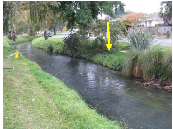
Figure 5b. The Tennyson Street reach in April 2011. The true right bank (arrowed) has slumped significantly
