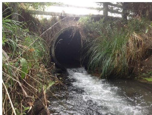
Photo 3. Downstream end of road culvert (Sabys Road) immediately upstream of Site 2: Creamery Stream. The culvert was perched and may present as a barrier to fish passage.
