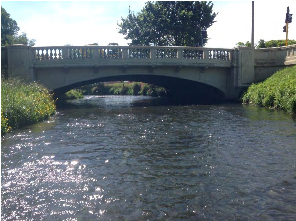
Avon River at Carlton Mill Corner (Site 25), looking upstream.
