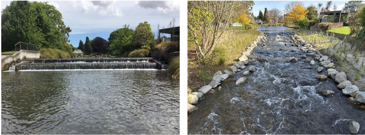
Figure 9: Mona Vale weir, in 2020 prior to remediation (left) and in 2023, after remediation to enhance fish passage (right).
