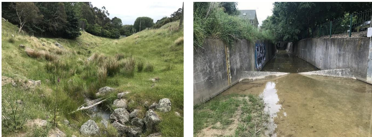
Figure 8: Site 10 (Sibleys Drain), showing the fish sampling reach (left) and downstream concrete-lined reach (right) identified as a fish barrier.
