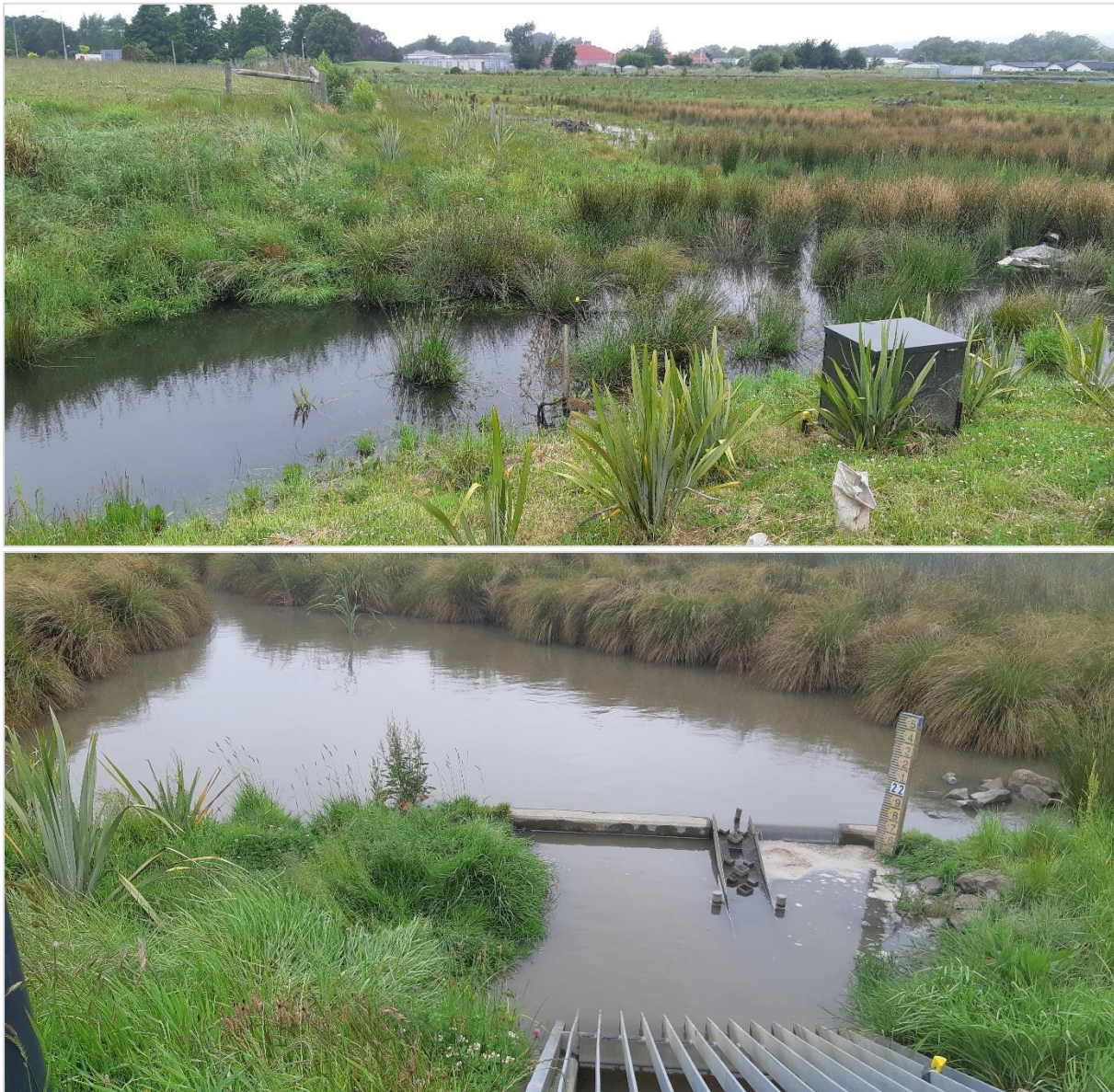
Figure 3-5: Curlett wetland inlet (top) and outlet (bottom). Photos taken 28 November 2021 (the day after Event 4). Note water is more turbid at the outlet than the inlet.
