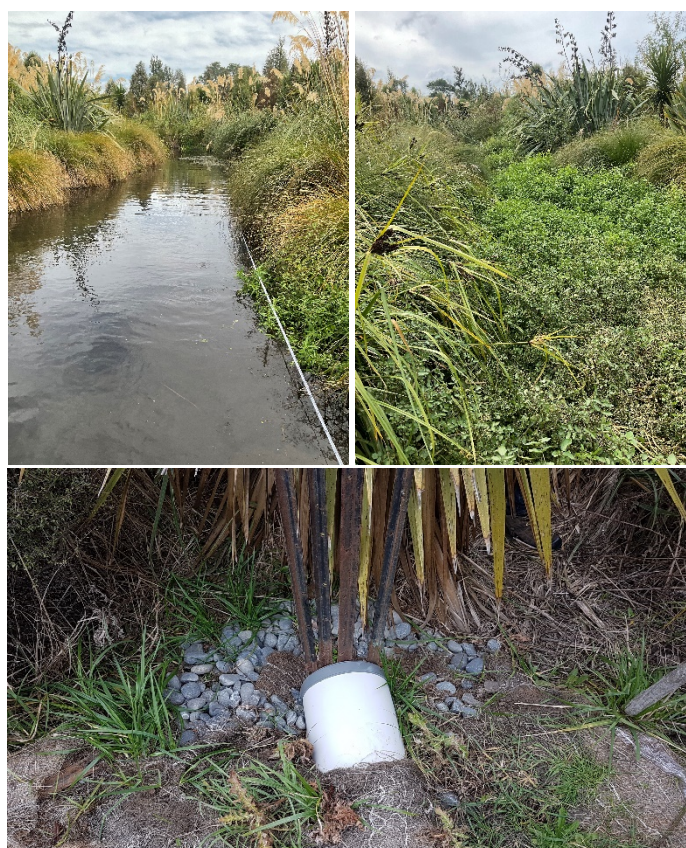
Photo 3. Site R1 view looking upstream (top left) and downstream (top right); construction-phase stormwater discharge pipe (bottom).
