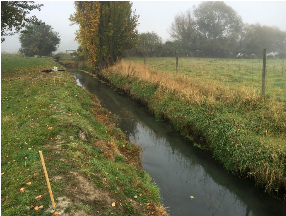
Figure 16: Site 4, view upstream from bottom of the reach.
