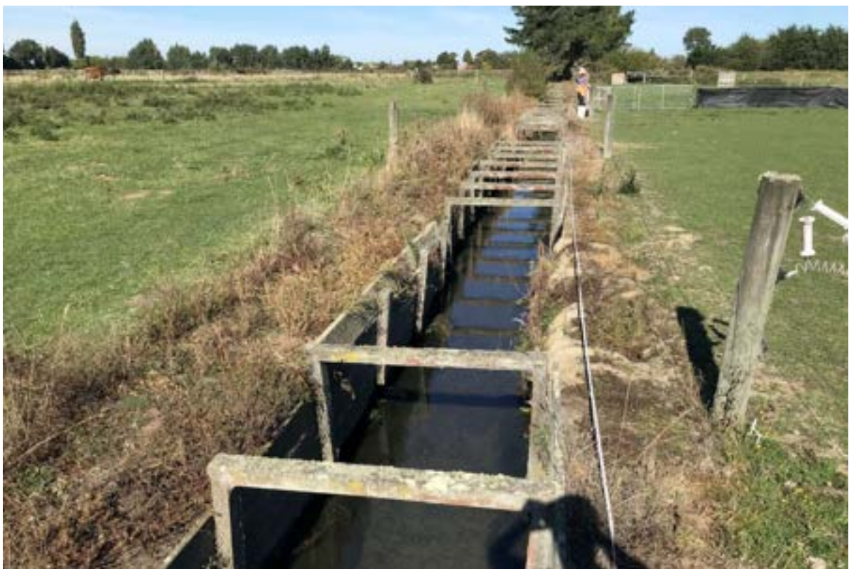
Figure 14: Site J1 (Johns Drain at 888 Main North Rd) – downstream looking upstream.
