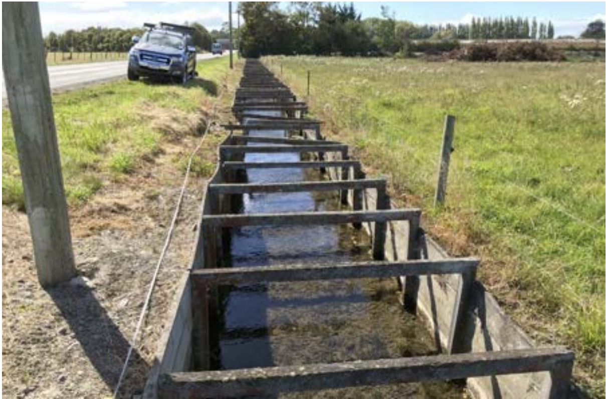
Figure 13: Site W1 (Wilson's Drain at Main North Rd) – upstream looking downstream.
