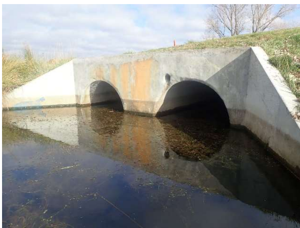
Figure 9: Inlet culverts to the pond system.
