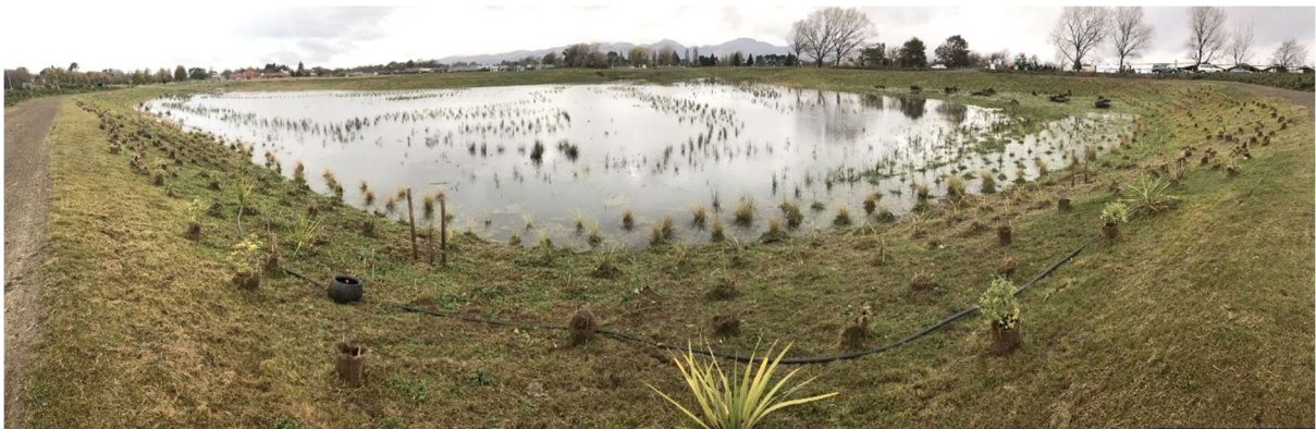
Figure 41: Curletts Basin after rainfall in May 2020.
