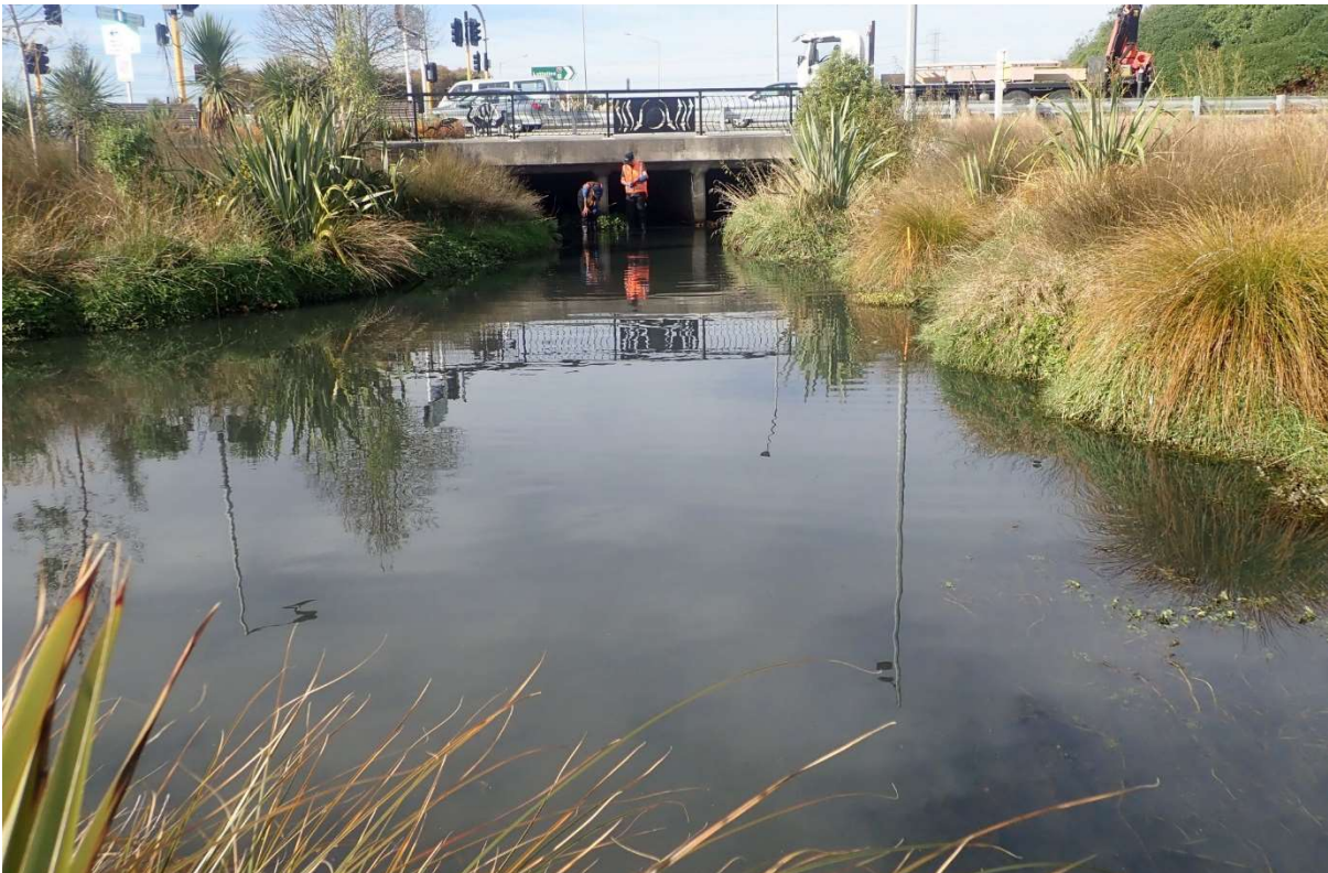
Figure 12: Site O2 (Linwood Canal / City Outfall Drain) – upstream looking downstream.
