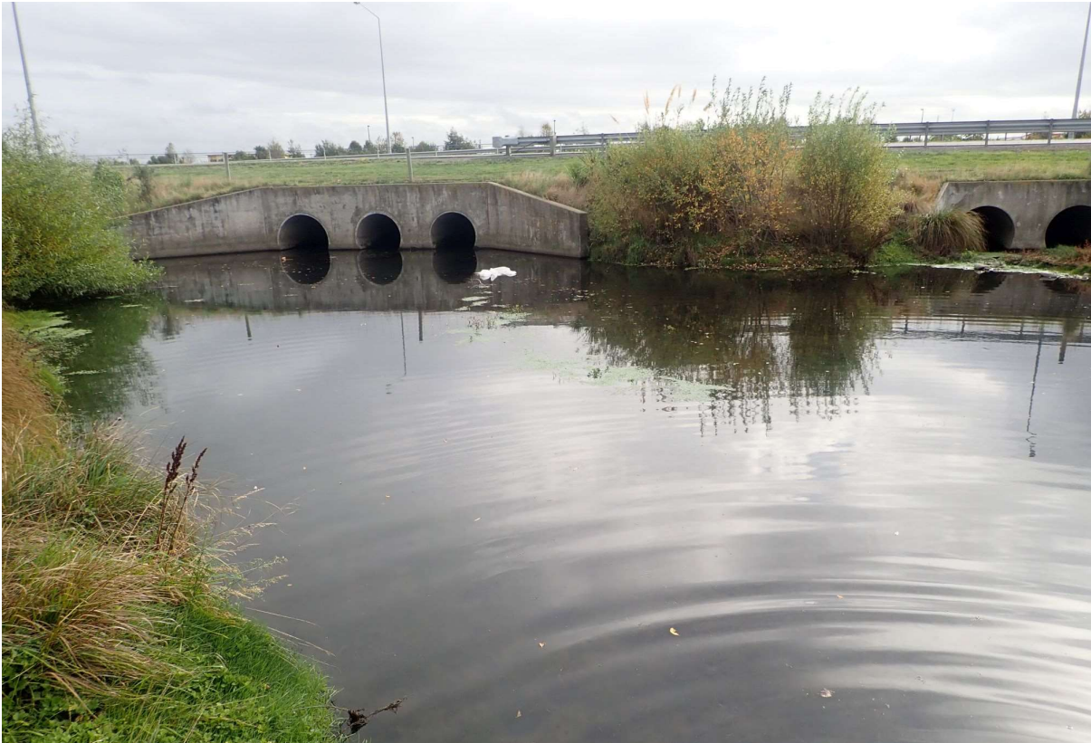
Figure 5: Site H14 (Curletts Road Stream at Southern Motorway) - downstream looking upstream.
