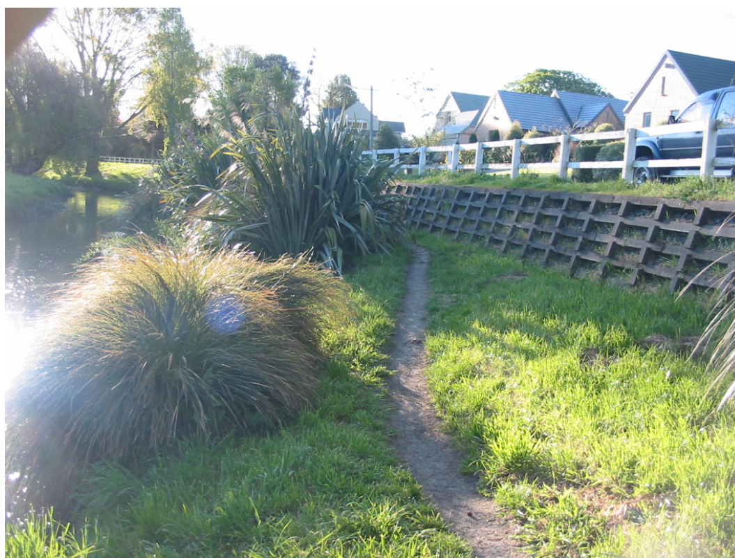
Figure 6. An example of a floodable terrace which provides vegetative fish cover during base flow, but hydraulic capacity and fish refuge during flood flows. The vegetation cover along should be more continuous than depicted here to provide ecological value.
