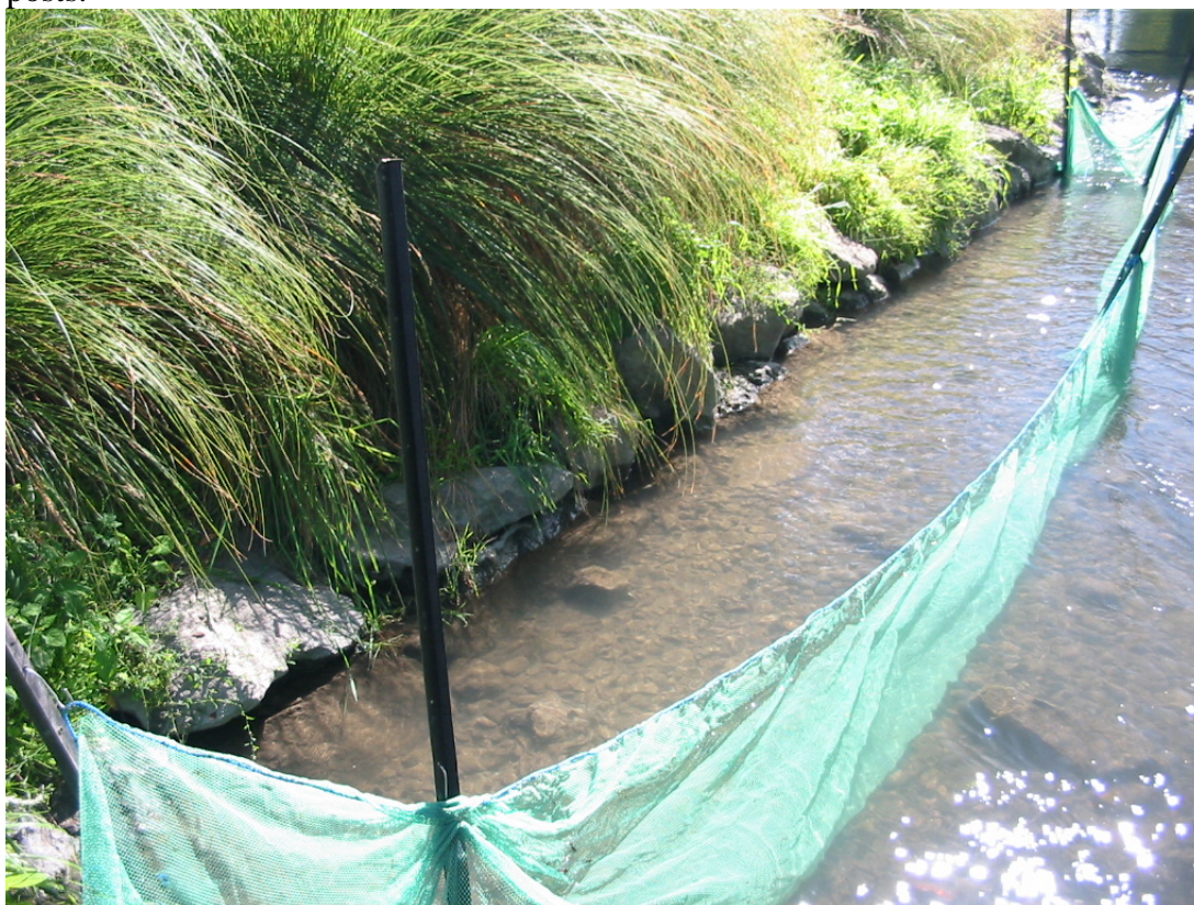
Figure 2. Netted bank treatment at Site 2, downstream of Malcolm Avenue.
