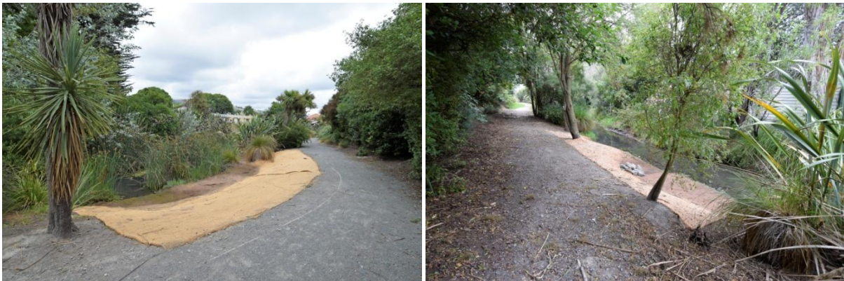
Figure 1. Two views of the Steamwharf Stream restoration area showing initial stabilisation work on the riparian margins between the recreational track and the waterway, January 2018. Photos: S. Orchard.
