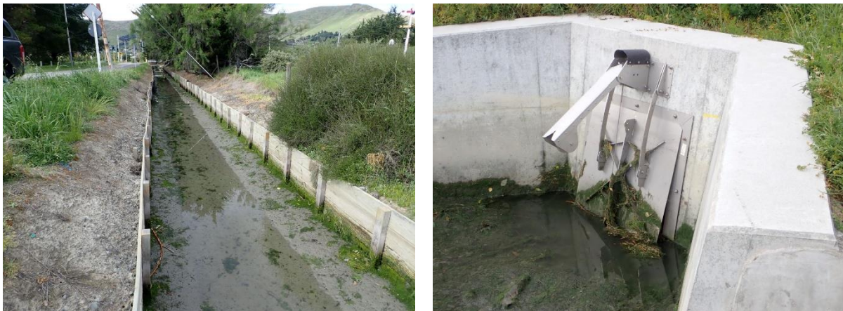
Figure 2: Truscotts Stream Branch (left) and its fish-friendly tide gate (right).
