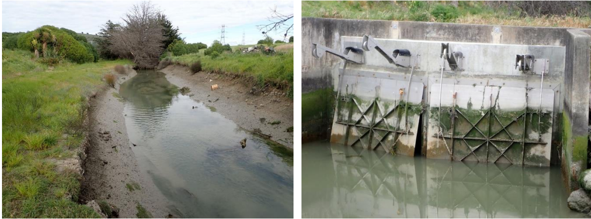
Figure 4: Avoca Valley Stream (left) and its fish-friendly tide gates (right).
