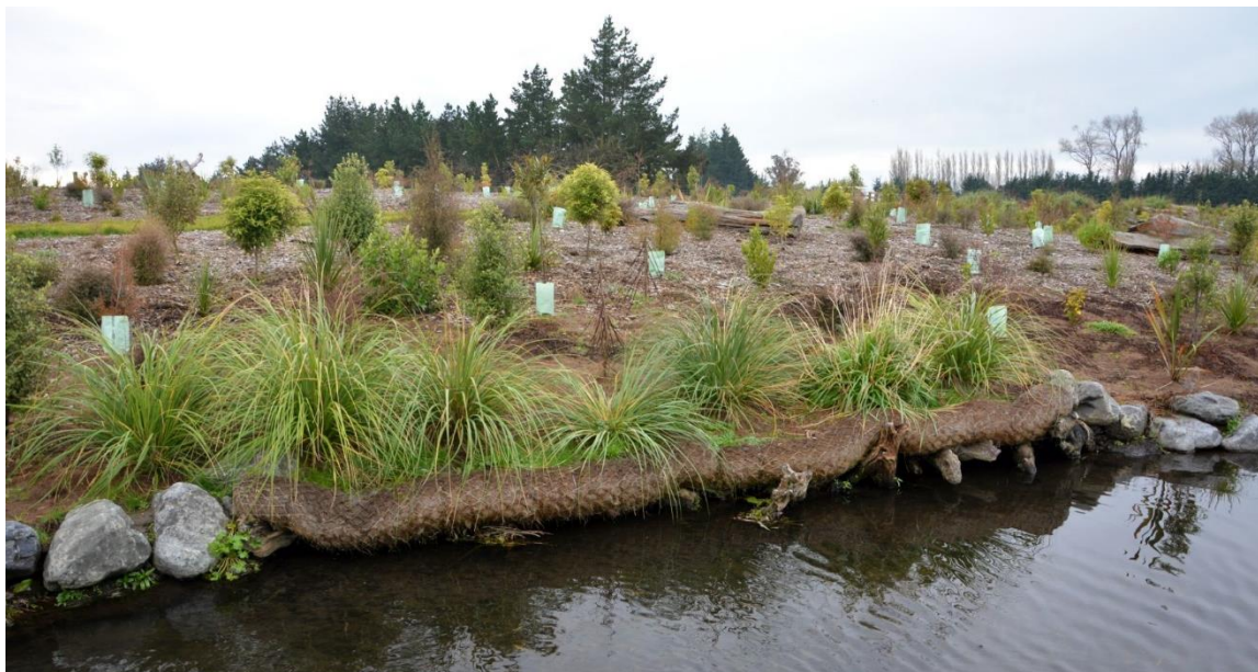
Figure 35: New native plantings and logs in the bank to provide fish habitat in the recently-realigned and enhanced section of Kā Pūtahi Creek (Site 11).
