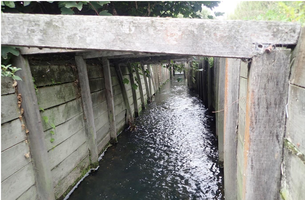
Figure 5: Site 12 (Horners Drain) - downstream end of reach looking upstream.
