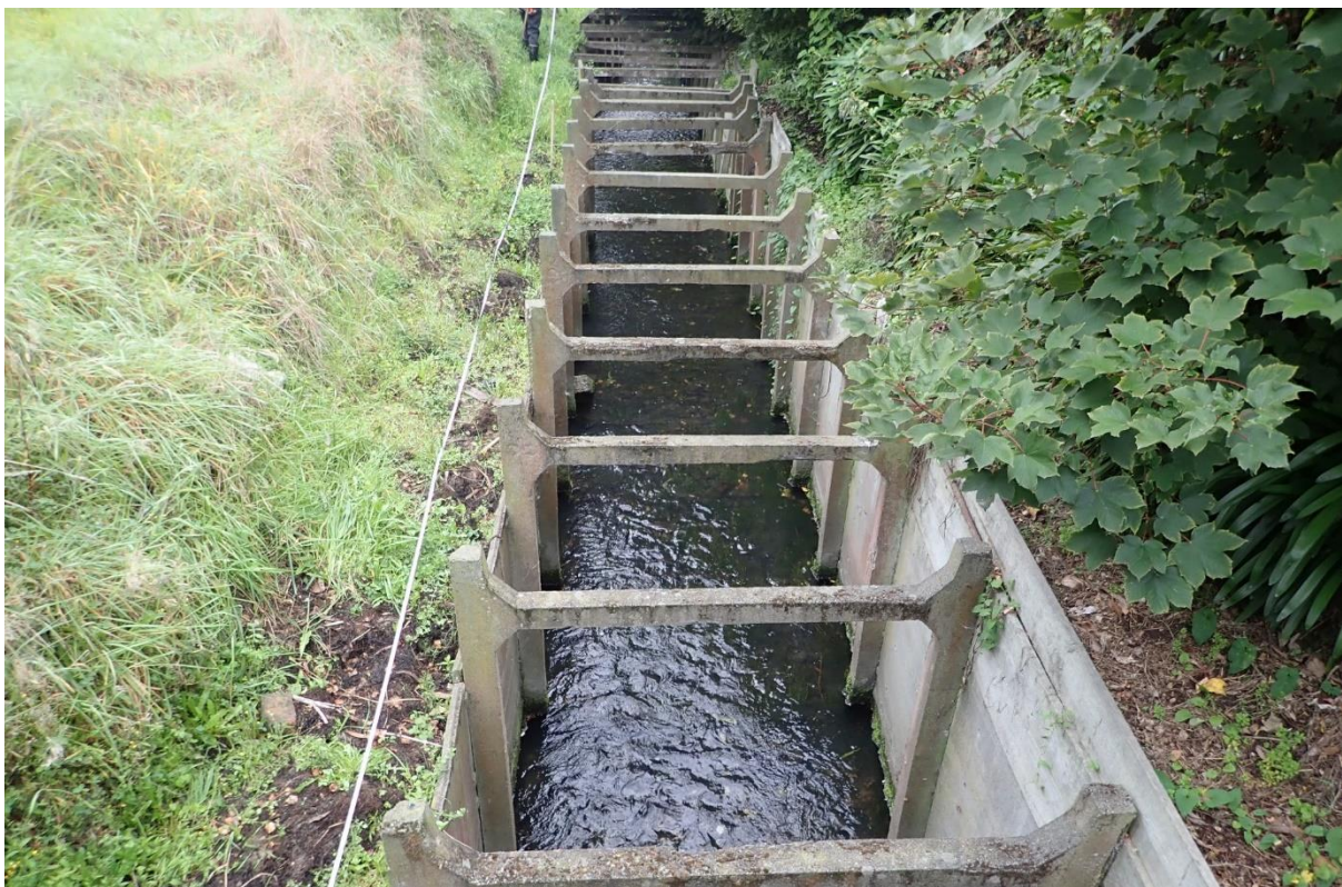
Figure 6: Site 12 (Horners Drain) - upstream end of reach looking downstream.
