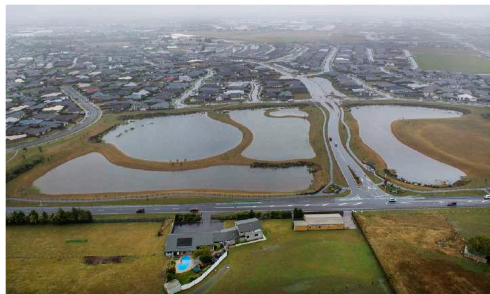
Awatea Basin flood Detention facilities. This services the new Wigram Skies subdivision and retrofits parts of Hornby March 2014
