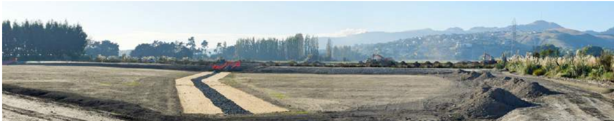
Eastman wetland under construction next to Henderson Basin and Sparks Road
