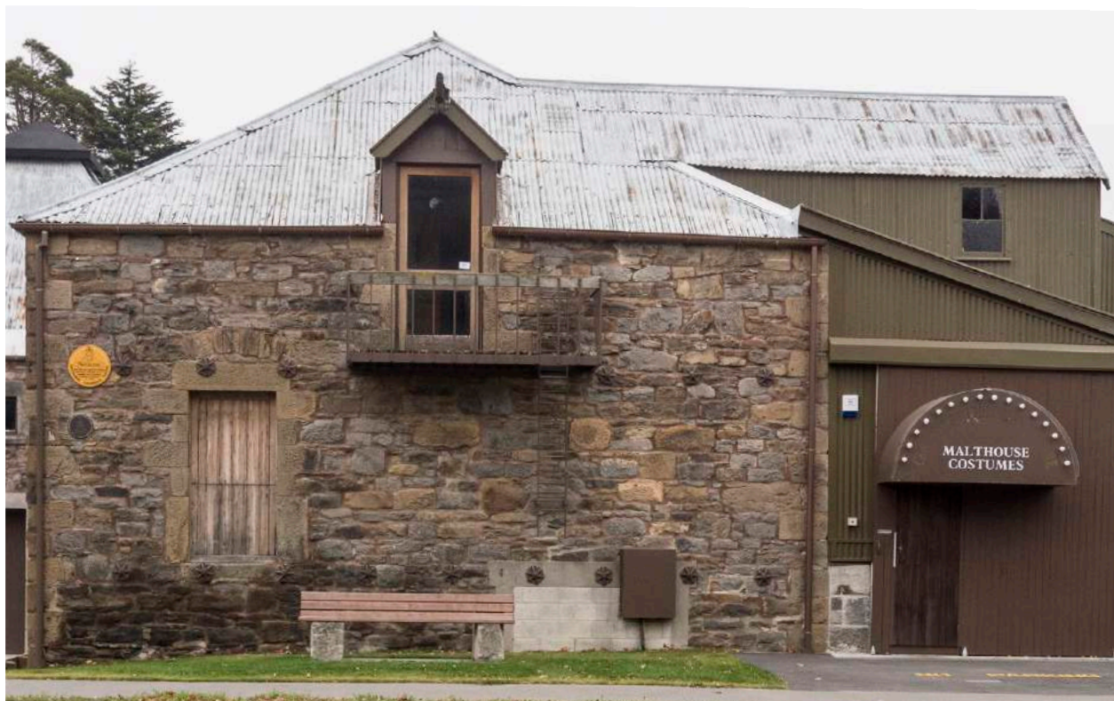
Malthouse beside the Ōpāwaho / Heathcote River
