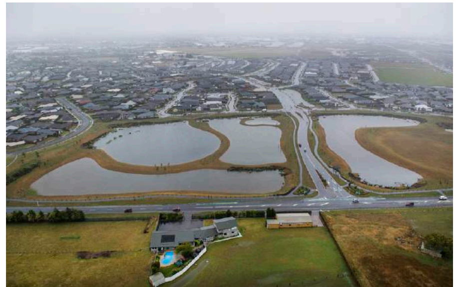
Ngāi Tahu, Wigram Skies subdivision, soakage and detention basins
