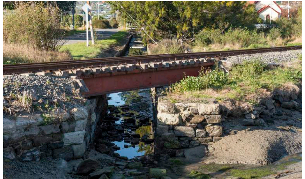
Stone lined drain, Ferrymead
