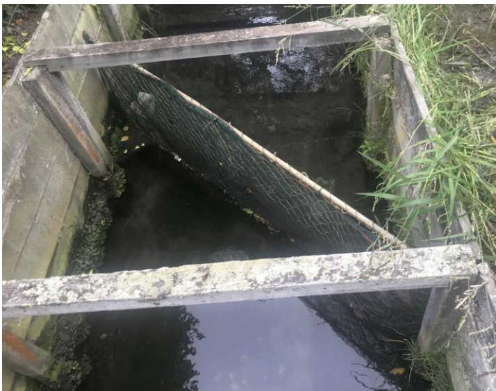
Example of a 'fence' type fish screen.
