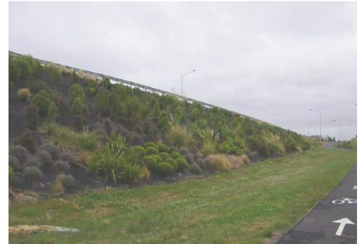
AFTER - Cycleway, swale and native embankment planting along motorway
