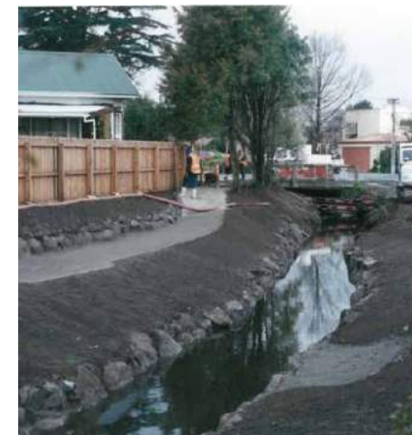
DURING CONSTRUCTION - Dudley Creek
