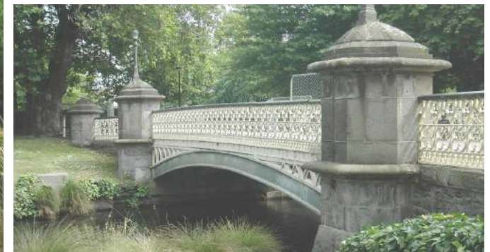
Victoria Street Bridge, Ōtākaro / Avon River
