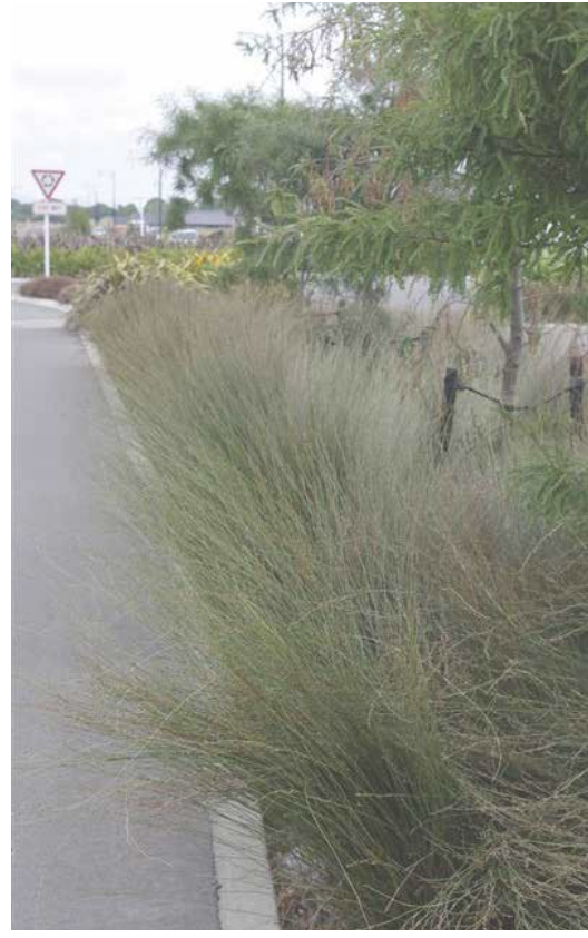
Native planting in swale in a new subdivision
