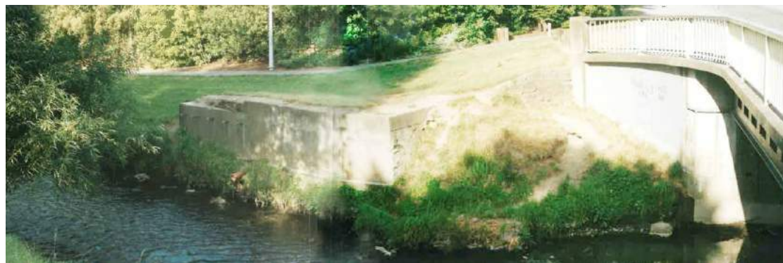
BEFORE - Old bridge abutment
