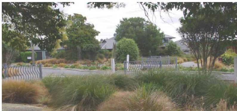
Enhanced walkways, road narrowing, swale and native planting along Papanui Stream, Proctor Street
