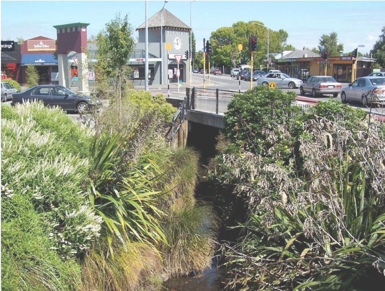
Waterway enhancement to carpark in suburban centre, Hills Road, Dudley Creek
