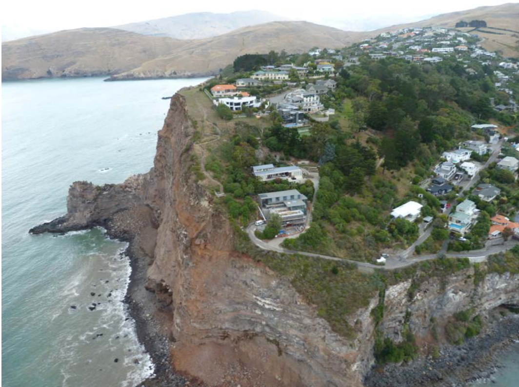
Figure 13A Whitewash Head following the 22 nd February 2011 earthquakes but before the 13 th June 2011 earthquake. Photograph taken by M. Yetton.
