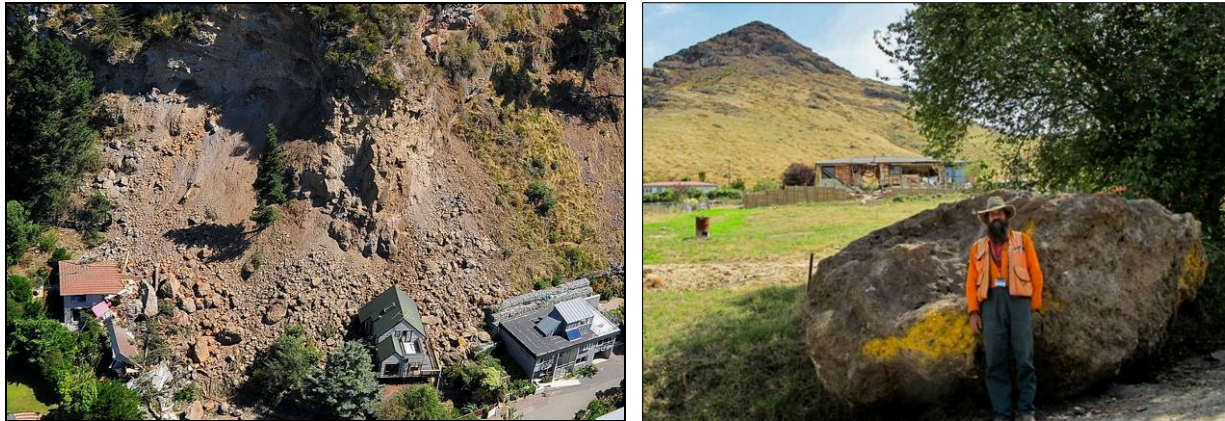
Figure 2 Illustration of the difference between cliff collapse with countless boulders (left, Raekura Place, Redcliffs) and rockfall where the location of each boulder can be precisely located (right, Rapaki Bay). Differences in what data can be collected about the two types lead to differences in how they are analysed to determine life-safety risk. The illustrated rockfalls occurred in the 22 nd February 2011 earthquakes. Photographs by G. Hancox (left); D. Barrell (right), GNS Science.
