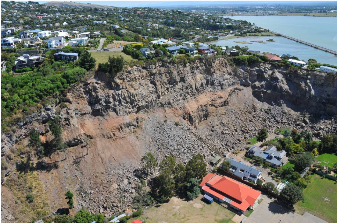
Figure 10 Redcliffs following the 22 nd February 2011 Christchurch Earthquake. Photograph taken by G. Hancox, GNS Science.
