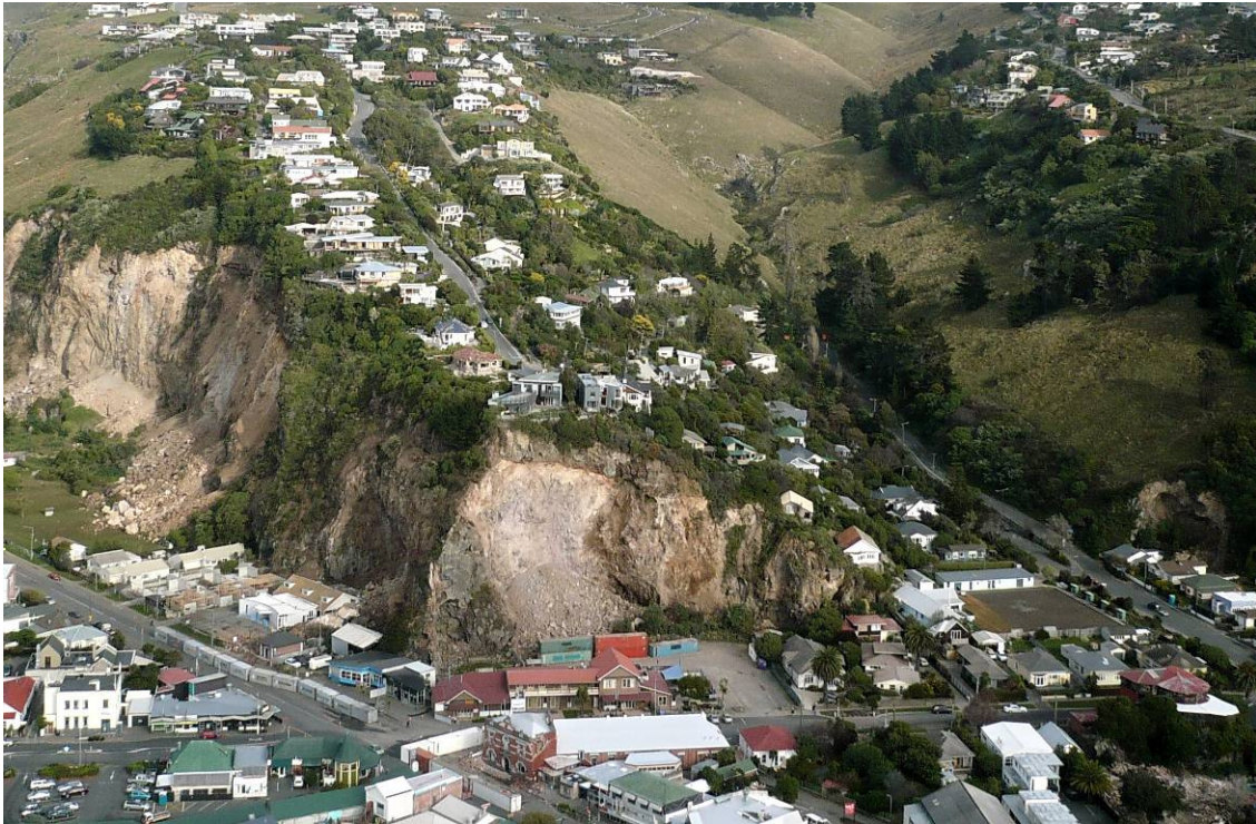
Figure 12 Nayland Street (foreground) and Wakefield Avenue (left) following the 13 th June 2011 earthquake. Photograph taken by C. Massey, GNS Science.
