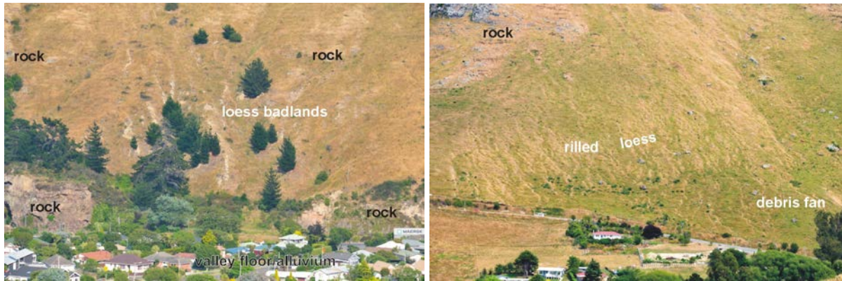
Figure 8 Loess deposits commonly have a distinctive geomorphic expression and erode to form bad-lands topography, as at Wakefield Street (left) (Grid Reference 1580400/5175300), or more commonly rills and terracettes, such as at Rapaki (right) (Grid Reference 1573900/5172000). Note also the large boulders lying on the surface and the break in slope to the debris fan on the right.
