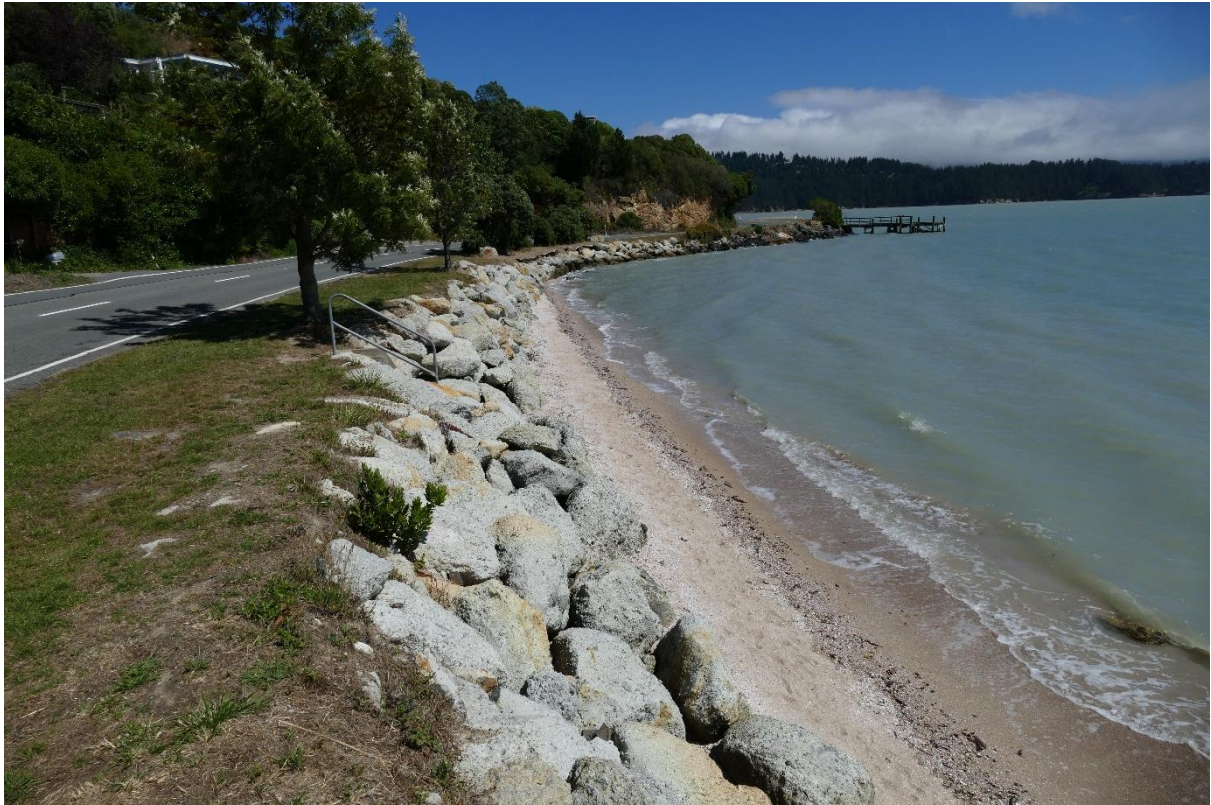
Figure G19 Rock revetment protection along road reserve in Charteris Bay (Area B in Figure G16)
