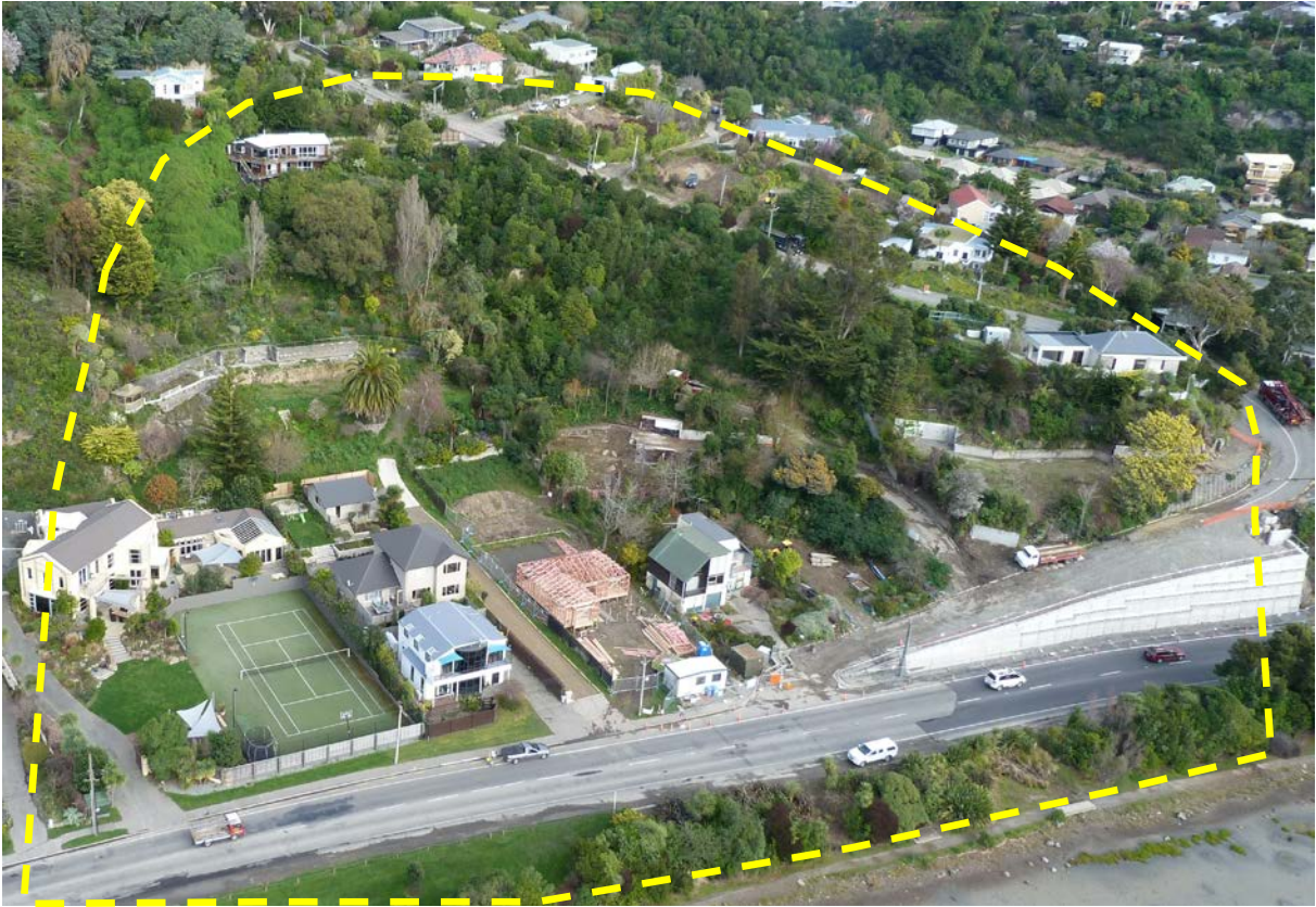
Figure 3 Aerial view, looking west, of the Maffey's Road assessment area. The approximate extent of the assessment area is shown by the yellow dashed lines, the actual mapped extent of the assessment area is shown on Figure 2). Photograph taken by M. Yetton (2013).
