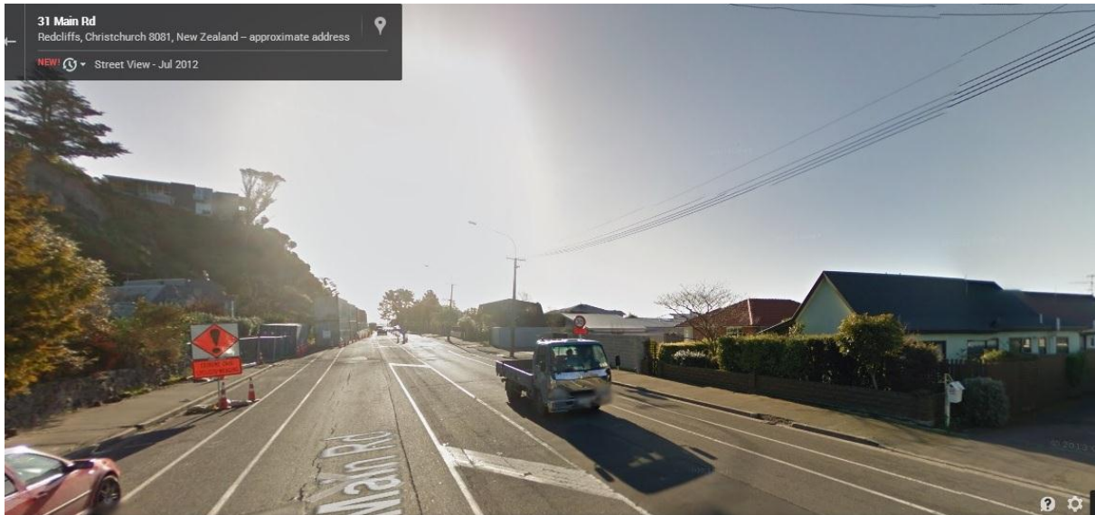
Figure A1.3 View northwest along the Main Road section assessed for Redcliffs (image taken from Google Earth).
