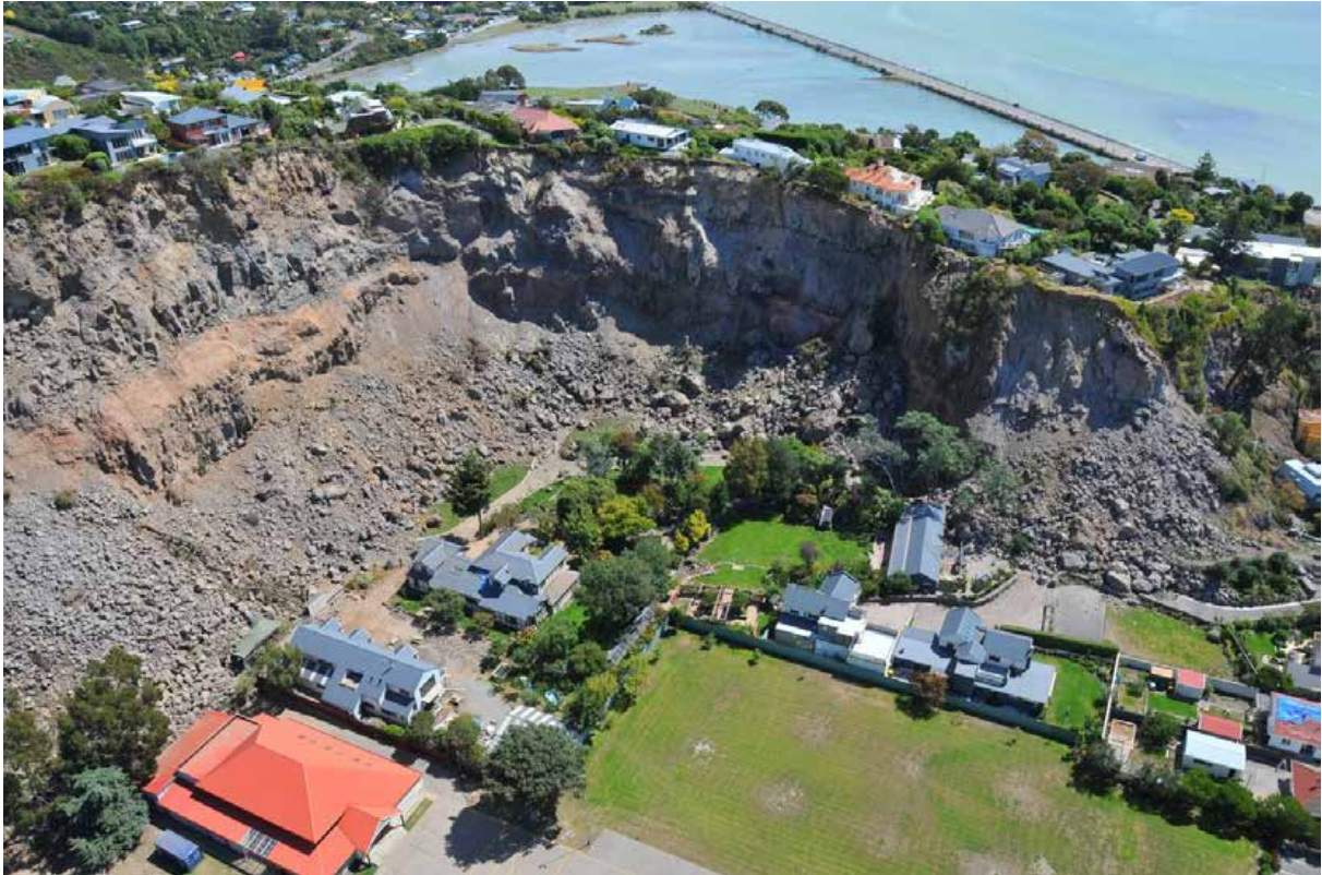
Figure 7 Aerial view of the Redcliffs mass movement area after the 22 February 2011 earthquakes and before the 13 June 2011 earthquakes. Photograph taken by G. Hancox.
