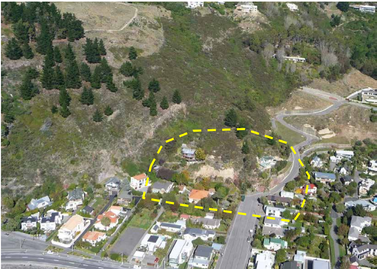
Figure 3 Aerial view of the Cliff Street mass movement study area number 6 (within the yellow dashed line), looking south.
