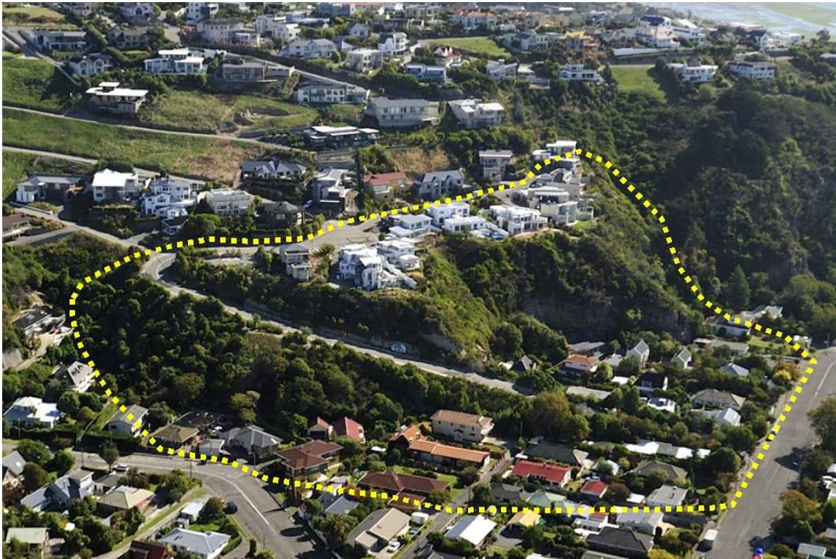
Figure 3 Aerial view of the Defender Lane mass movement study area looking west.
