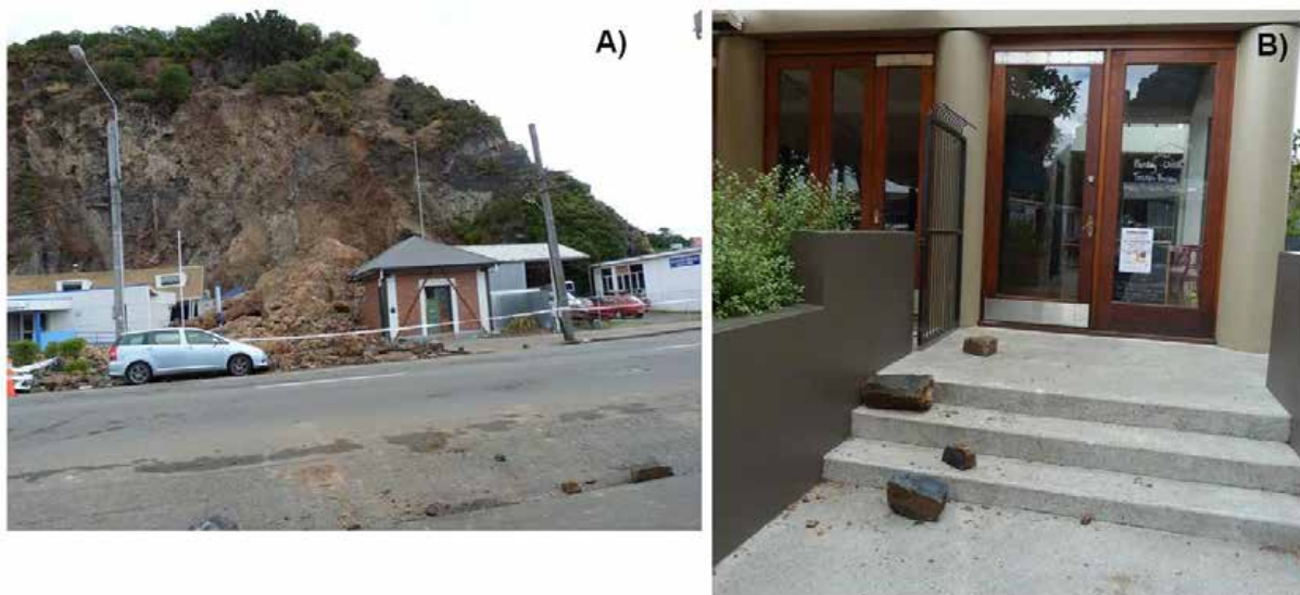
Figure A1.2 Debris avalanche at the northern end of Richmond Hill site triggered by the 22 February 2011 earthquakes. A) Photograph looking west across Wakefield Avenue – note debris in the foreground and some debris has been cleared from the road. B) Photograph looking east from Wakefield Avenue, opposite photograph A) showing fly-rock debris. Photographs taken by M. Yetton.
