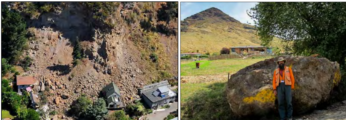
Figure 2 Illustration of the difference between debris avalanches caused by cliff collapse (left at Raekura Place, Redcliffs) and rockfall (boulder roll) (right at Rapaki Bay). The large boulder in the foreground of the Rapaki view fell from the peak (Rapaki) in the background, passed through the home in the mid-ground, and came to rest on the foreground road, 60 m from the house. These landslides occurred in the main 22 nd February 2011 earthquake. Photographs taken by G Hancox (left); D Barrell (right), GNS Science.
