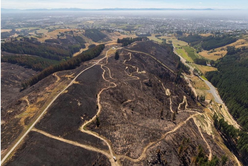
Damage to commercial forest and Chch Adventure Park cycle tracks above Cashmere Valley (April 2017).
