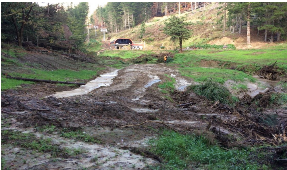
Run-off from fire break (20 April 2017).
