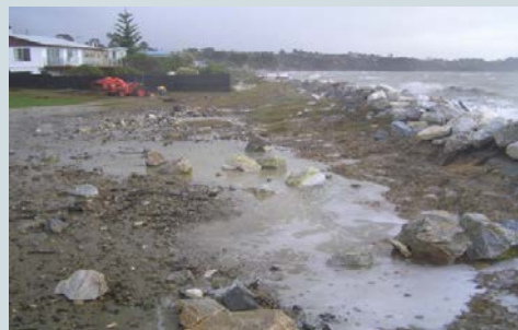
Photo credits: (left) Mapua foreshore; (right) Ruby Bay rock revetment after a wave-overtopping event (both E Verstappen, Tasman District Council).
