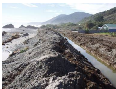
Figure 38: Wash out of a gravel barrier on the west coast of the South Island
