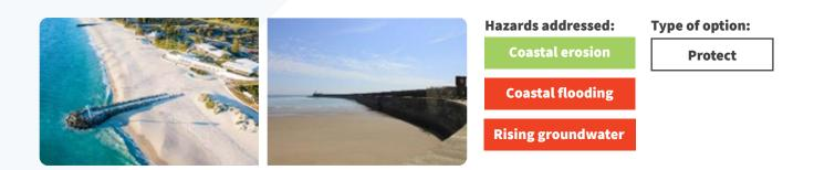
These structures are built perpendicular to the shoreline out into the sea to catch sediments that are transported along the coast by longshore drift. By trapping sediment, the beach is widened and therefore more wave energy can be dissipated and erosion can be reduced.
