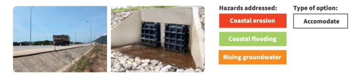
Flood proofing infrastructure such as roads, wastewater, stormwater and drinking water networks, and telecommunication infrastructure may involve modifying existing assets or designing new or replacement assets to withstand coastal hazards.
