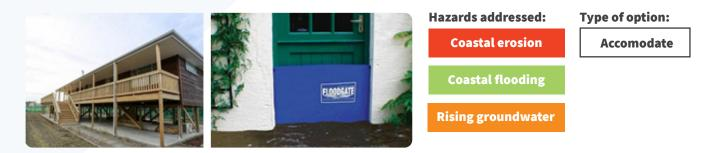
Flood proofing buildings is achieved using two main methods: wet or dry flood proofing. Wet flood proofing involves three main techniques; allowing water to enter and leave structures easily to minimise structural damage, using flood resistant materials, or elevating structures and utilities, while dry flood proofing ensures buildings are watertight up to a certain level. Flood proofing measures may be temporary or permanent.
