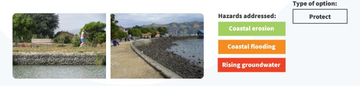
Armouring hardens the edge between land and water. This may take the form of seawalls, revetments, gabion baskets, reno mattresses or cobble beach armouring.
