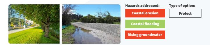
These structures protect low-lying areas from inundation by building an elevated barrier. They are usually earthen, covered with vegetation and in the context of coastal hazards are parallel to the shore of low-lying coastlines and rivers.
