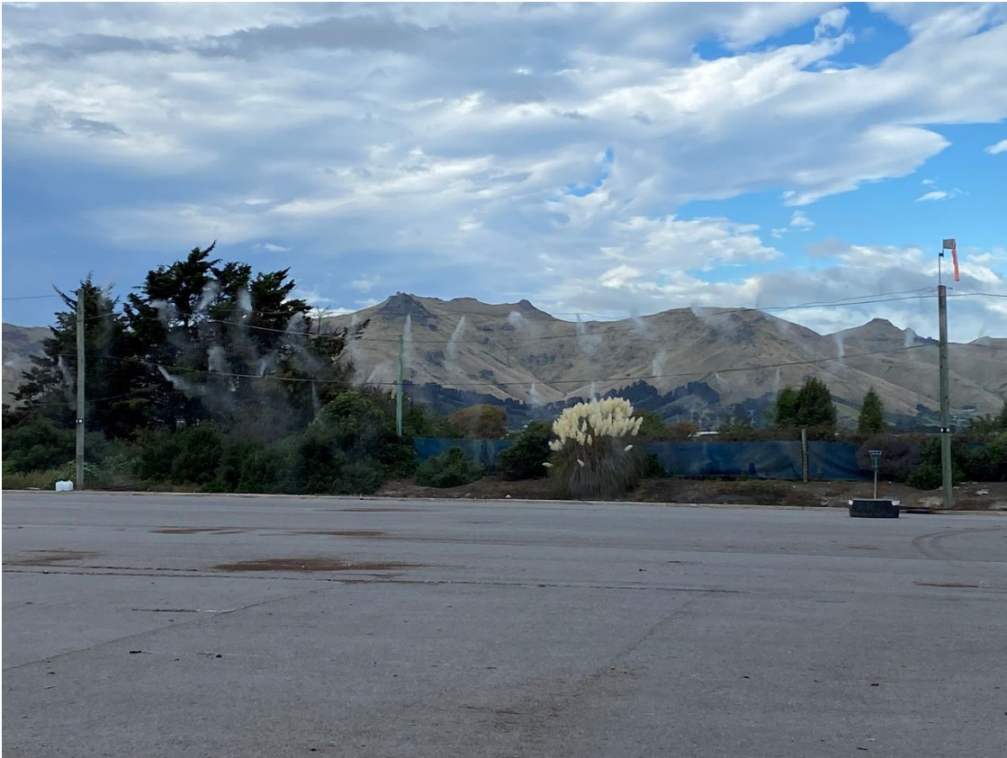
Figure 3: Misting line on southern boundary
