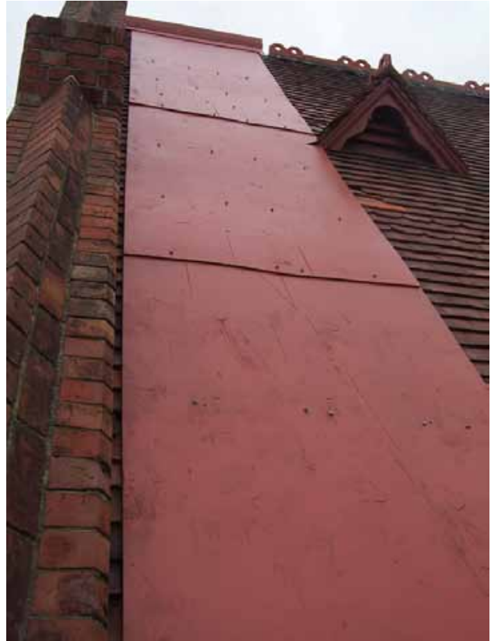
Painted plywood provides weatherproofing.
