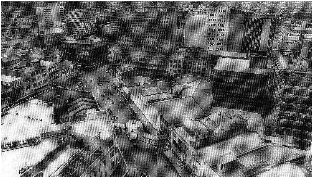
Figure 78. Looking towards the Square from the south-east, 1983: the Cathedral spire is obscured by the BNZ building. High Street has become a pedestrian mall with an overbridge. Rice G W, Christchurch Changing an Illustrated History, p149
