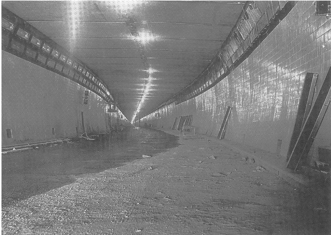
Figure 8. Road tunnel to Lyttelton nearing completion. Opened on 27 February 1964, it was designed as a toll tunnel (New Zealand's longest) but became toll-free in 1979. Christchurch Star
