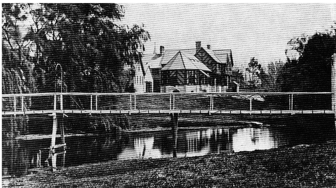
Figure 119. Antigua Street suspension bridge and a section of the original Public Hospital buildings, 1872. Lamb RC, p108, Britenden Collection CHAC/CM
