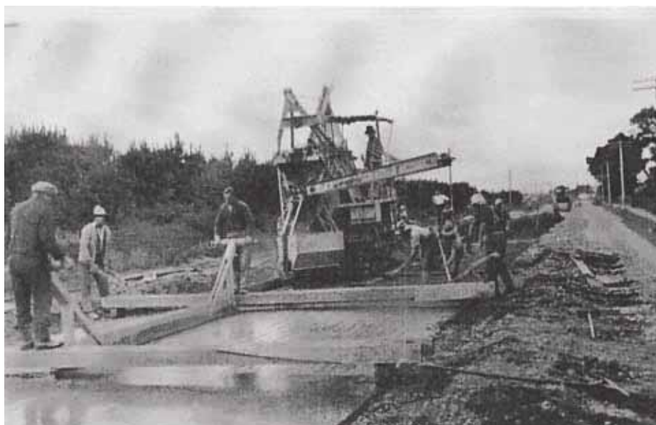
Figure 13. Road construction, Sockburn. 1930s. ATL collection
