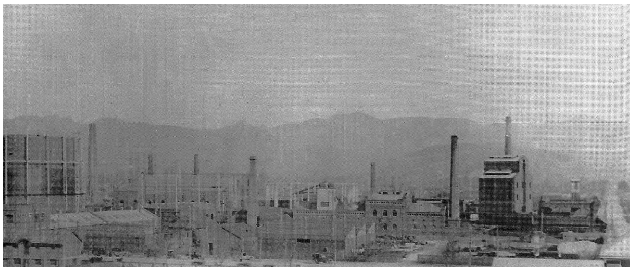
Figure 34. The Christchurch gasworks, c. 1930. Coal gas was produced here from 1864 until 1982, after which the site was completely cleared, including large quantities of contaminated soil. S. W. Perkins photograph, CHAC/CM 873
