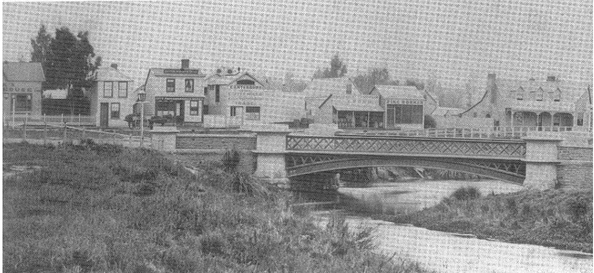
Figure16. The second Victoria Street bridge, 1865. Probably the earliest iron-and-stone bridge in New Zealand, it is now preserved as the Hamish Hay Bridge in Victoria Square. Dr A.C. Barker photograph, CM41
