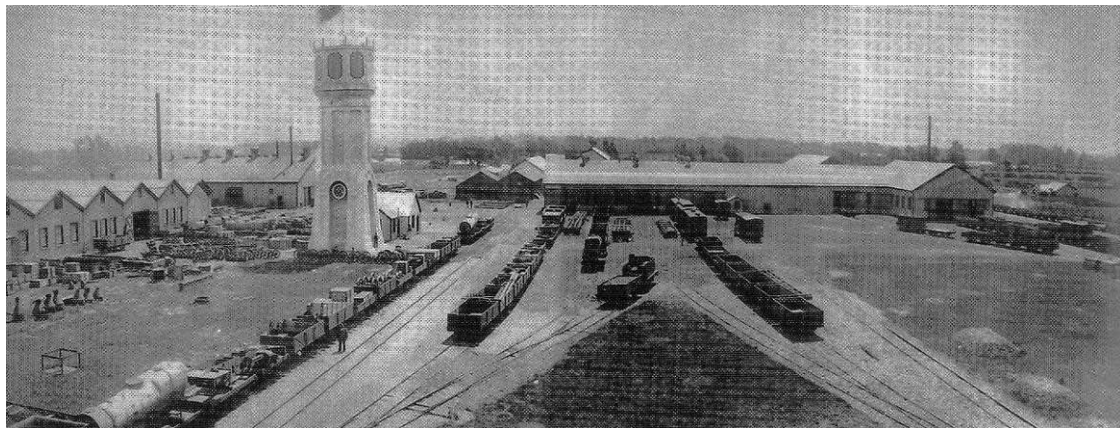
Figure 12. Addington Railway Workshops, soon after completion of the water tower (1883), one of New Zealand's earliest reinforced concrete structures. The workshops became one of the city's biggest employers in the late nineteenth century, and produced New Zealand's first locally designed steam locomotive (W192) in 1889. French collection, CHAC/CM 931
