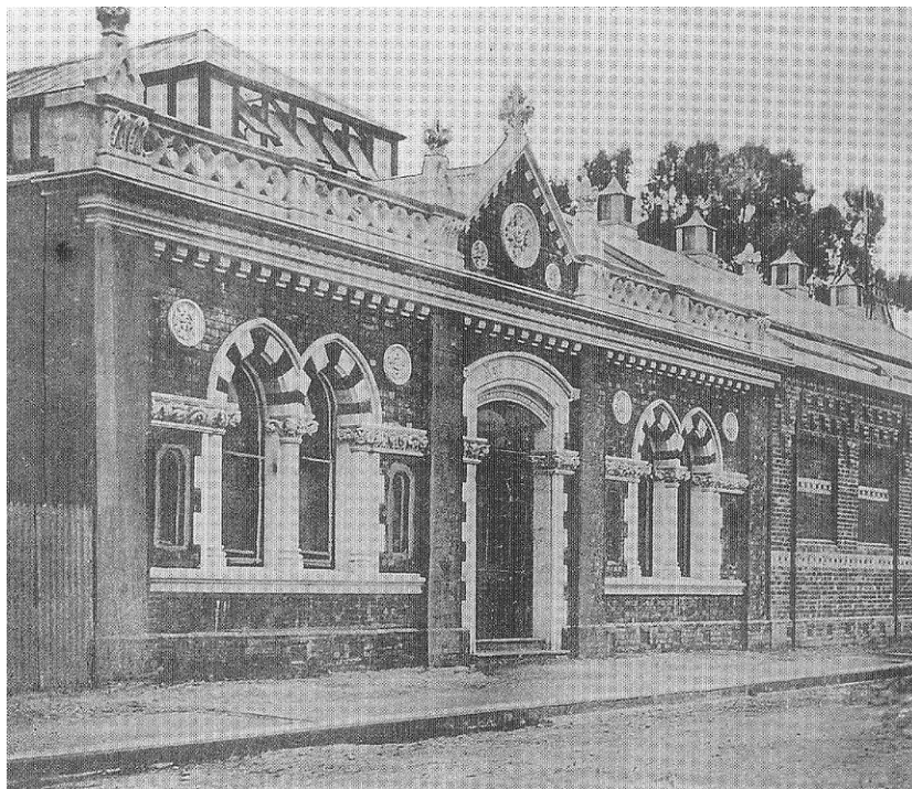
Figure 103. Art Gallery, Durham Street in 1890. The Canterbury Society of Arts raised the money to build the original gallery (right) by public subscription, and added another wing (left) by 1897, when this photograph was taken. Although the building survives, some of its ornamentation has been removed as an earthquake risk. Wheeler and Son photograph, CM 4828
