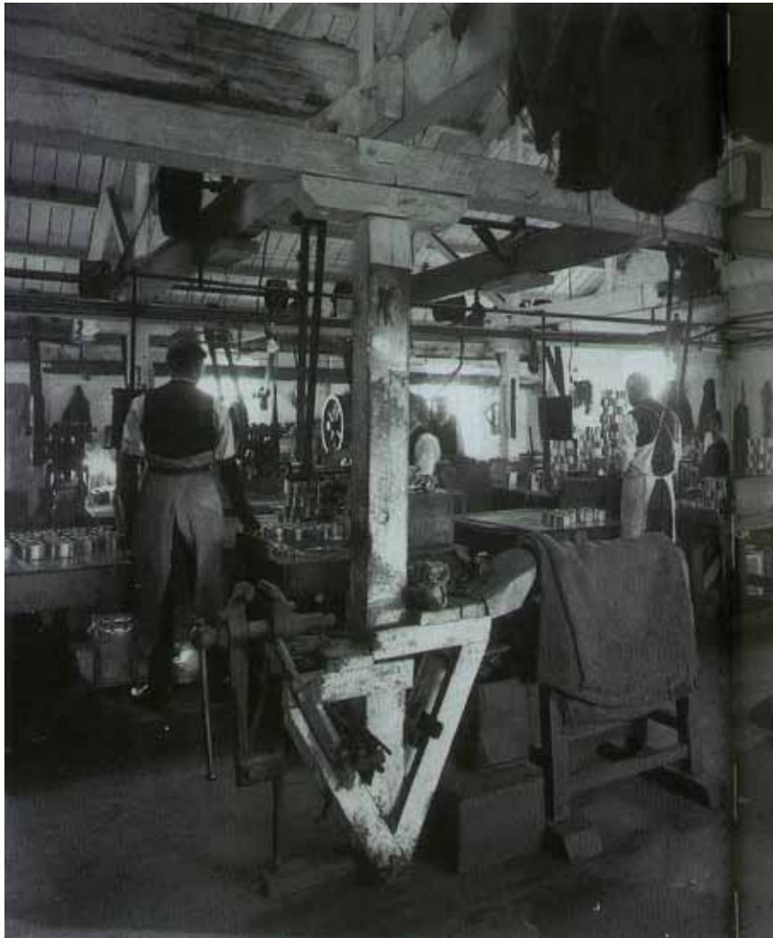
Figure 60. Christchurch Meat Co.'s canning plant. Alexander Turnbull Library 19429 1/1
