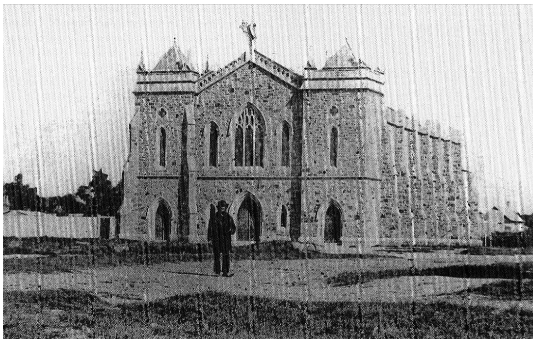
Figure 84. Durham Street Methodist Church, which opened on Christmas Day, 1864. This is the earliest-known photograph (probably taken soon after completion) of the first stone church on the Canterbury Plains, and one of the city's earliest Gothic Revival stone building. Rice GW, p 37, Britenden Collection, CHAC/CM
